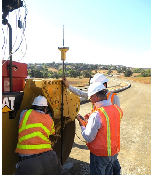
Figure E.2 - GPS Calibration Process.
