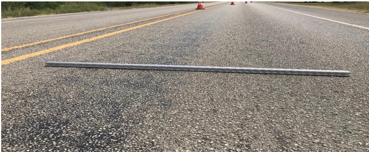
Figure A.17. Flushing in BU 181/SH 123 –Karnes County
