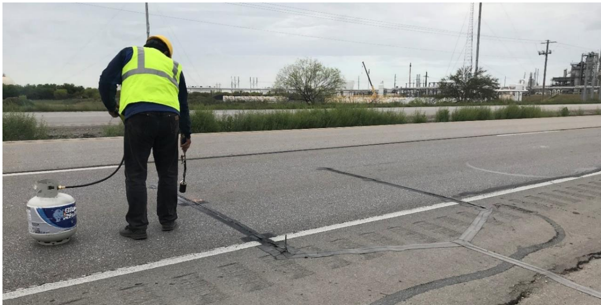
Figure 4.4. Portable WIM Field Installation in the Winter Time
