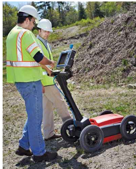
Figure 5: GPR system used for geotechnical investigation (trenchlesstechnology.com)
