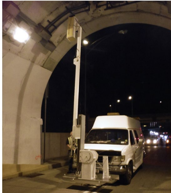
Figure 4: PennDOT is using a van-mounted GPR system to inspect tunnel walls [1].
