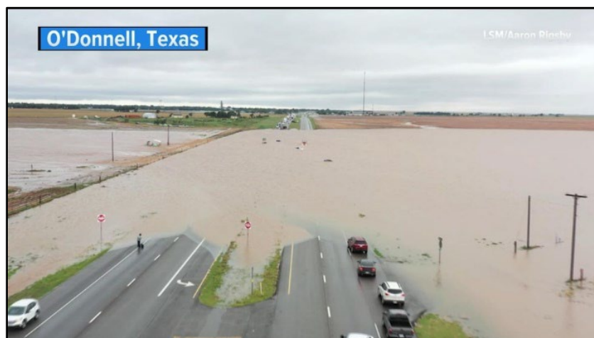
Figure B.26 Western Texas flash flood damage to a roadway in O'Donnell (ABC News, 2023)
