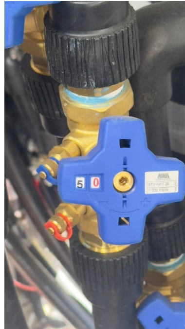
Manifold Balancing Valves
