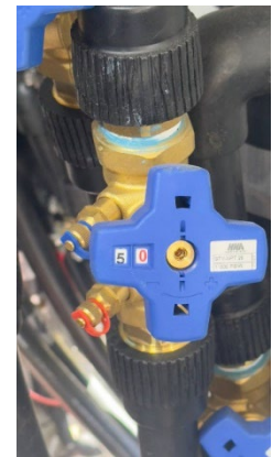
Manifold Flow setter
