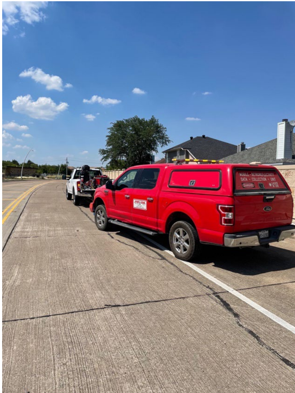
Figure 11: Traffic control during the ablation operations.
