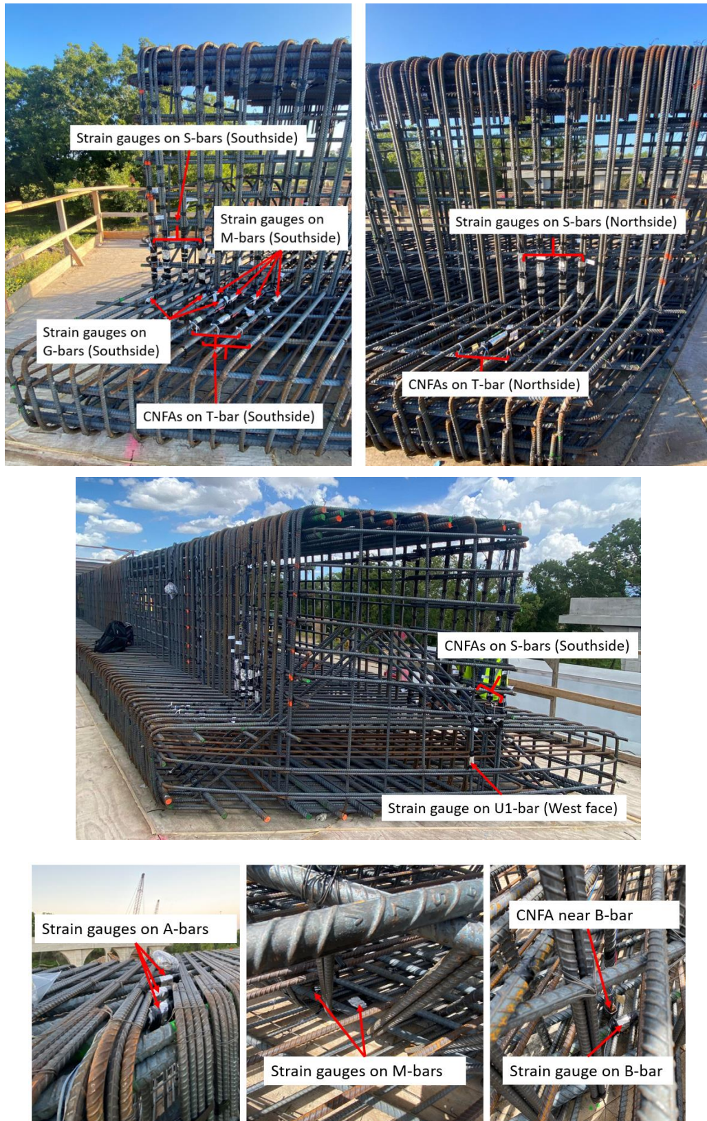
Figure A6.2. Strain Gauges and CNFA Instrumented on Bent Cap 2
