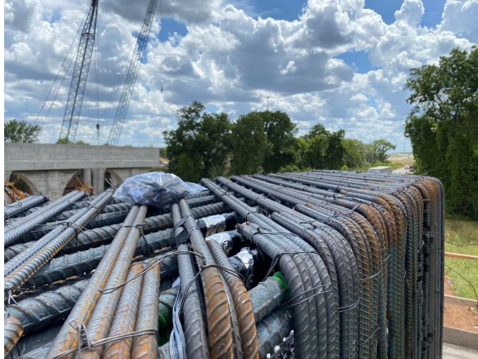
Figure 7.2. Rebar Congestion (S-bars), Bent Cap 2
