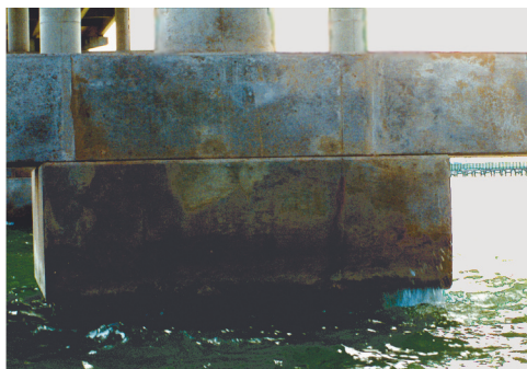
Figure 4 Even during calm seas, wave action attacks CPS anode margins at the bottom of the footers.
