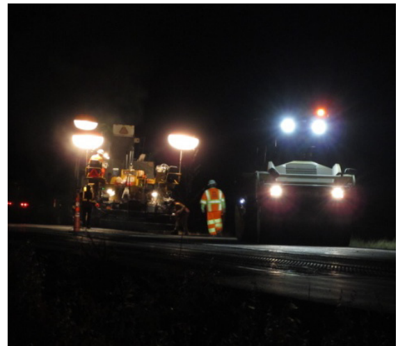
Figure 1. Paving Operation in Bryan/College Station, Texas.
