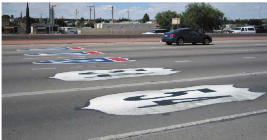
Figure 1. Example of In-Lane Pavement Marking Shields.
