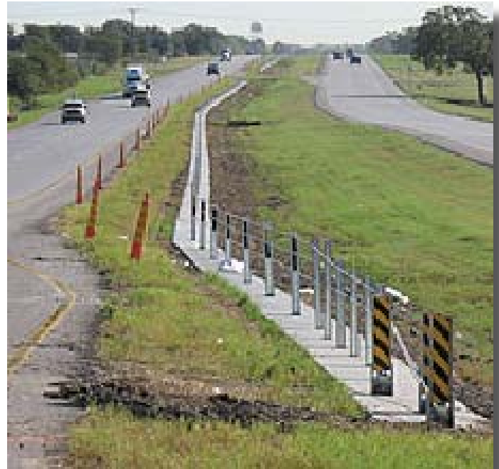
Cable Barrier with Concrete Mow Strip.
