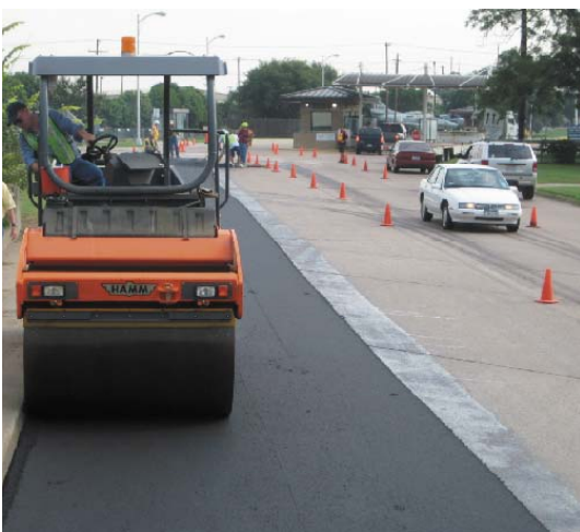
Figure 1. Placement of the CAM Mix on Pumphrey Drive, Fort Worth.
