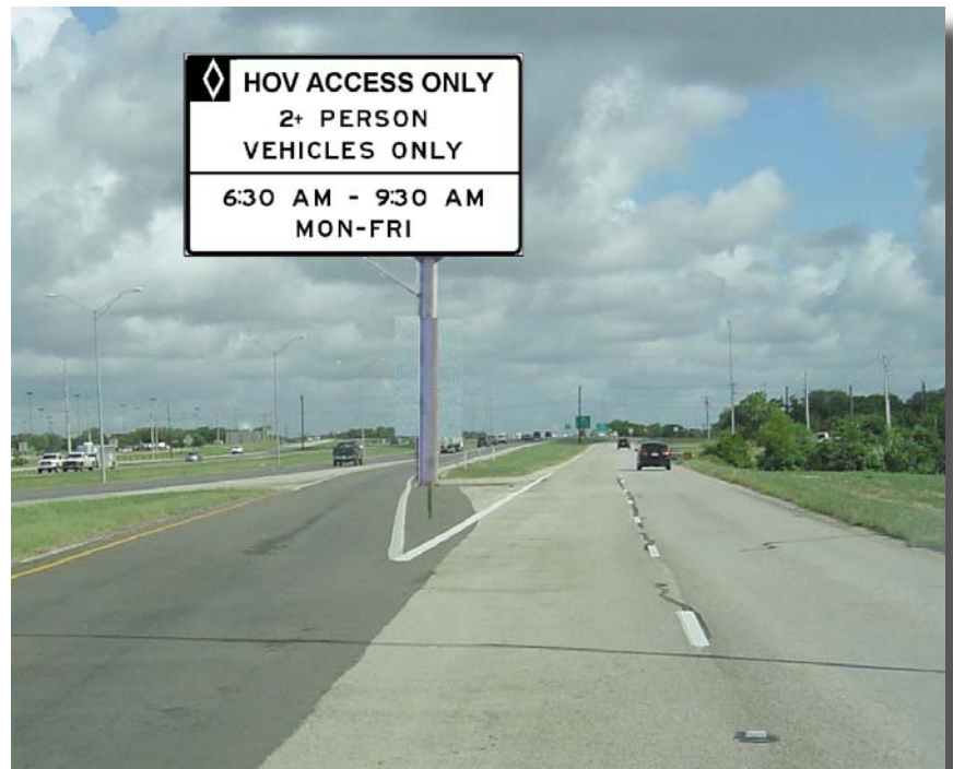
HOV Access Ramp
