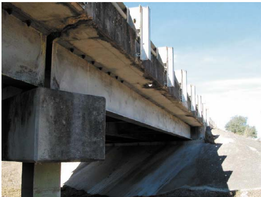
Post-Installed Shear Connectors in Bridge Located Near Hondo, Texas.
