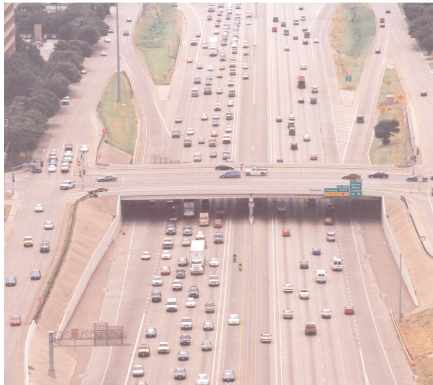
Figure 2. Limited access concurrent flow lanes along I635 (LBJ Freeway) in Dallas, Texas
