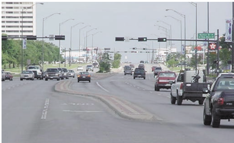
Figure 1. Raised median treatment along Texas Avenue in College Station, Texas
