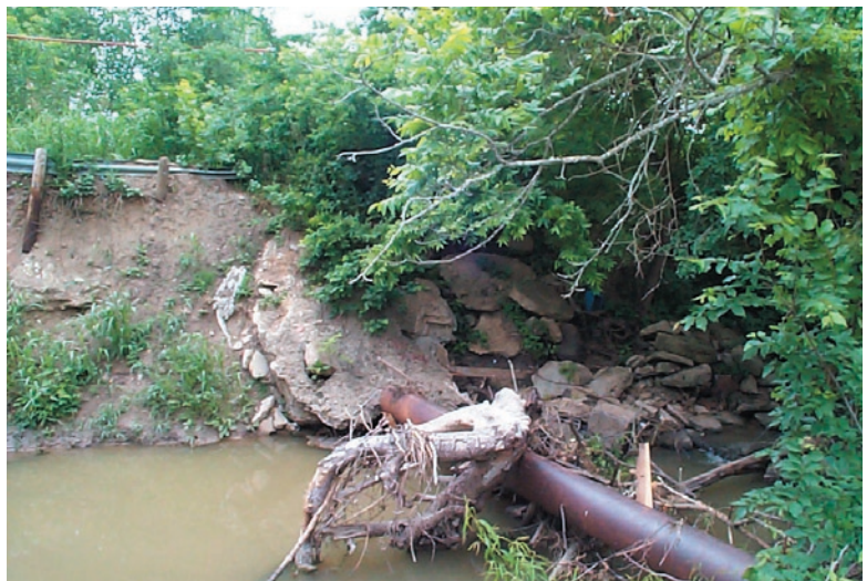
Figure 1. Guardrail posts exposed after erosion of the streambank/embankment. Abandoned pipe crossing the creek caught a lot of debris. (Photo taken in May 1999)
