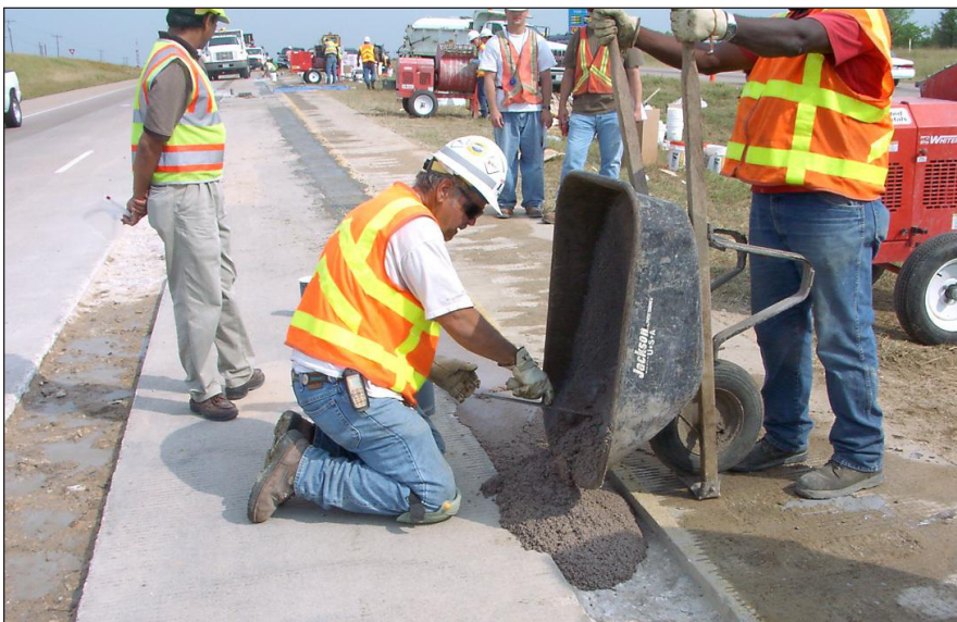
Figure 2. Placement of FlexPatch by Crews in Ft. Worth.
