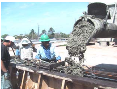
Fig. 5 Casting of I-Beam-B2
