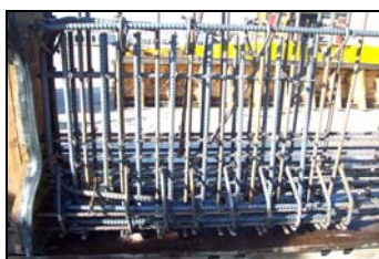
Fig. 2 End Zone Reinforcement in a Prestressed I-Beam
