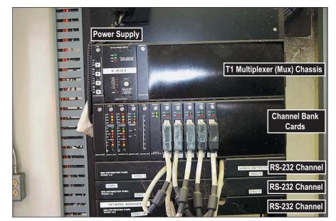
Figure 2. T1 Multiplexer and Channel Cards in a Typical Field Hub Installation.
