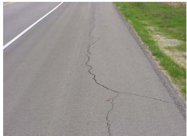
Figure 2: Longitudinal and Transverse Cracks on Paved Shoulders
