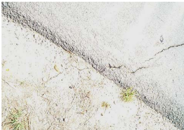
Figure 1: Shoulder Cracking of SH 108 Unpaved Shoulders (Transverse Cracks)
