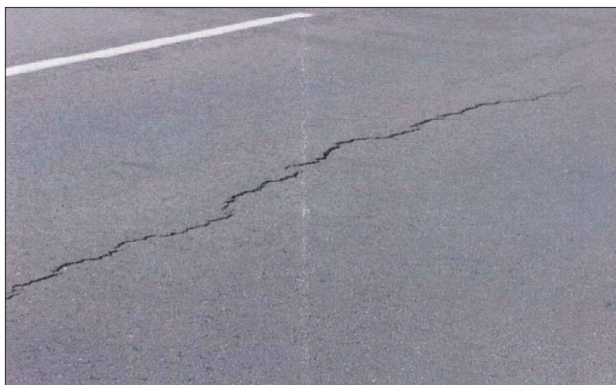
Figure 2. A Typical Shrinkage Crack of the Pavement Surface in the Vicinity of Trees and Other Vegetation.
