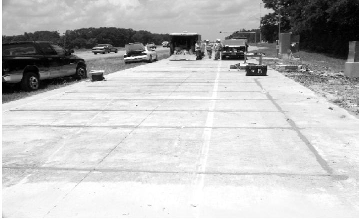
Figure 4. Sensor installation in New Waverly, TX.
