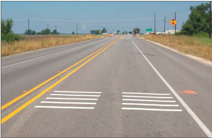
Figure 1. Typical Installation of TRSs.
