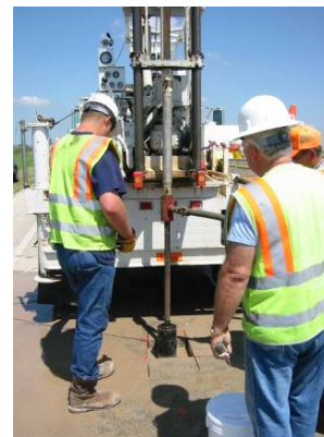
Fig. 6. Field installation at Bryan District SPS-8 Site
