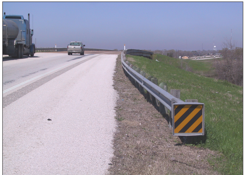
Figure 1. Example of a Roadside Safety Device in Use by TxDOT: The ET-2000 End Treatment.
