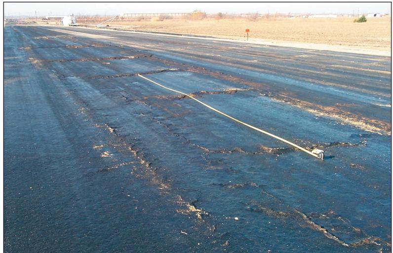
Figure 1. Vertical Heaves Generated during Construction of US 67 near Midlothian.
