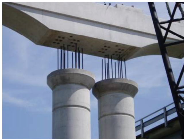
Figure 1 – Construction of Lake Belton Bridge Project using Grouted Vertical-Duct Connectors
