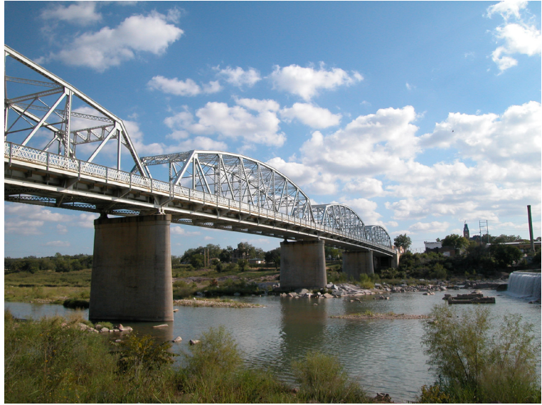
Figure 2: Case Study Bridge in Llano, Texas
