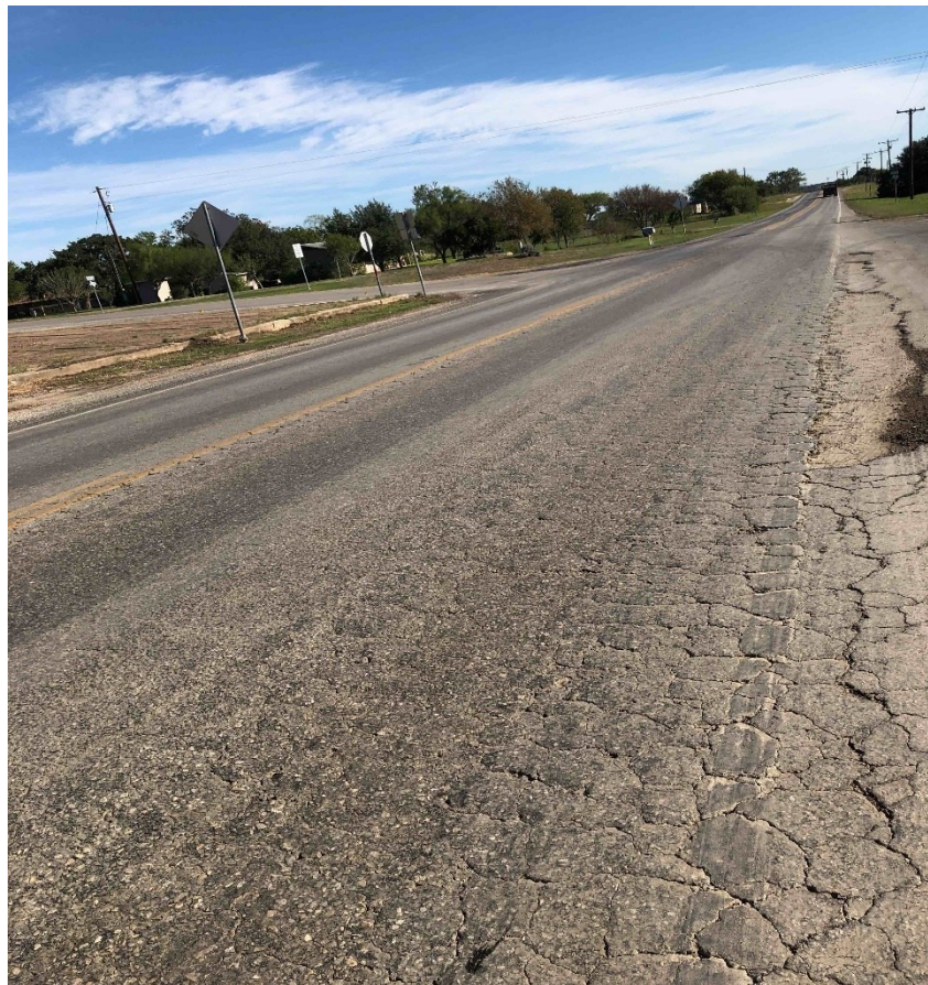
Figure 42. FM 81 Pavement Condition: Severe Wheel Path Fatigue Cracking.
