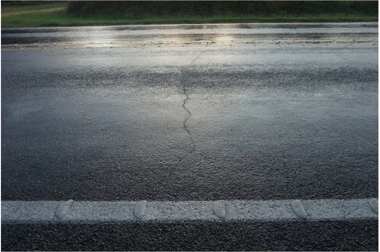
Figure 70. FM 99 Pavement Condition in October 2021: Transverse Cracking.
