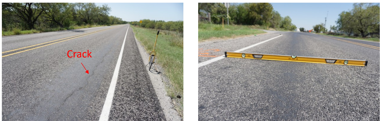
Figure 69. FM 99 Pavement Surface in September 2017: (a) Cracking and (b) Rutting.
