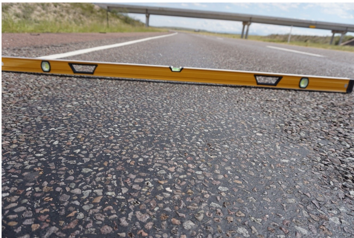
Figure 65. Pavement Surface Rutting on I-10.
