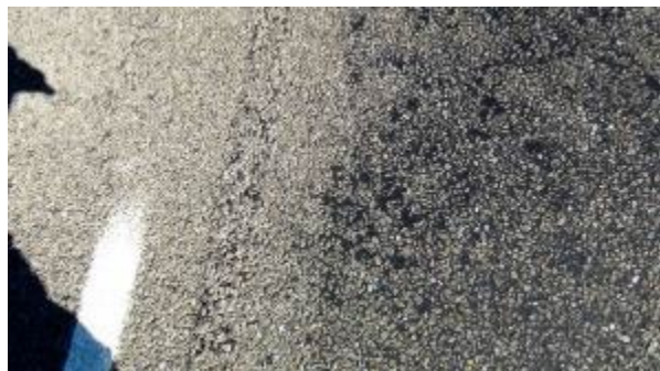
Figure A-529. SH0029-5, Inside WP.
