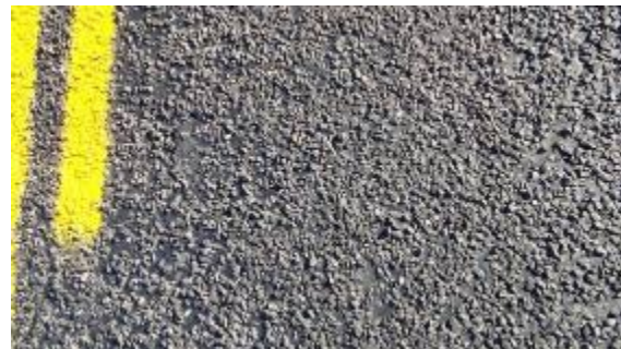
Figure A-884. SH0289-1, Inside WP.
