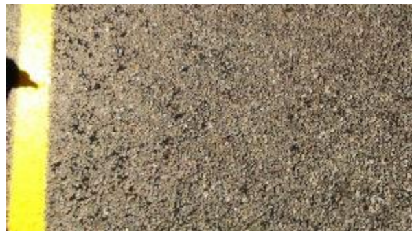
Figure A-473. SH0029-1, Inside WP.
