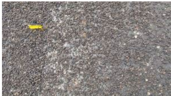
Figure A-353. SH0070-7, Inside WP.
