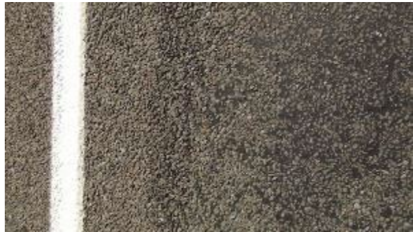
Figure A-541. SH0029-6, Inside WP.
