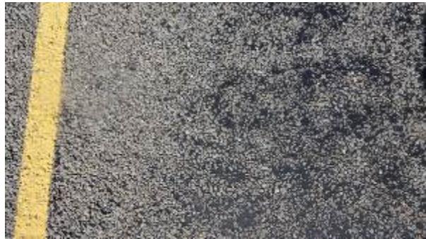
Figure A-509. SH0029-2, Inside WP.
