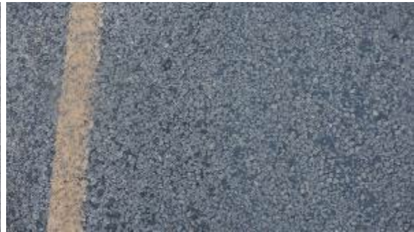
Figure A-88. SH0092-2, Inside WP.
