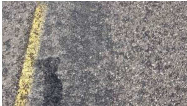
Figure A-365. SH0070-6, Inside WP.
