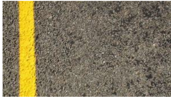
Figure A-477. SH0029-2, Inside WP.
