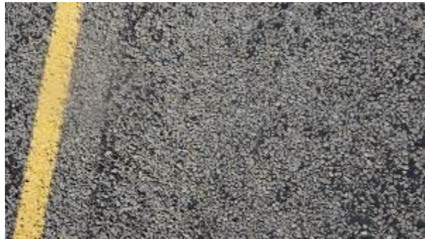
Figure A-517. SH0029-4, Inside WP.
