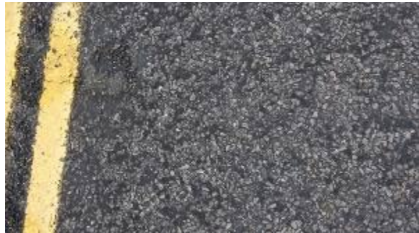
Figure A-914. SH0289-1, Inside WP.
