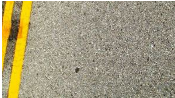
Figure A-872. SH0289-2, Inside WP.
