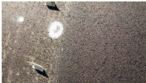
Figure A-521. SH0029-5, Inside WP.
