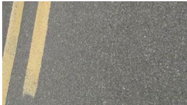
Figure A-329. SH0070-1, Inside WP.
