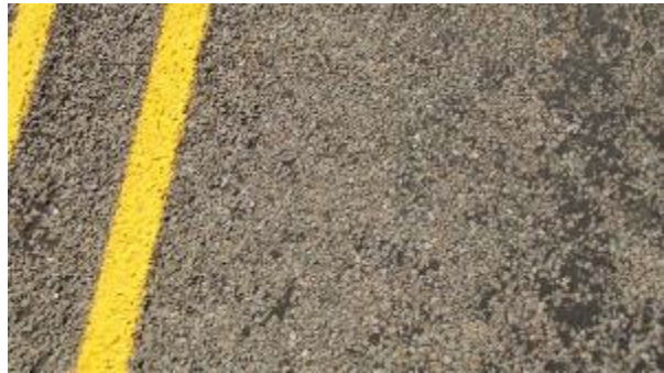
Figure A-493. SH0029-2, Inside WP.
