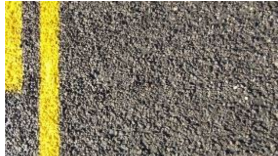
Figure A-888. SH0289-2, Inside WP.
