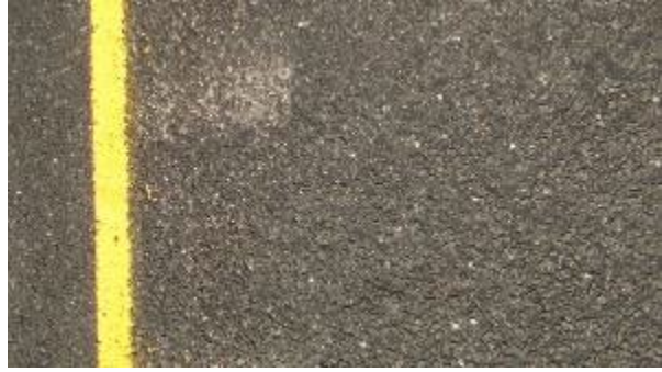
Figure A-910. SH0289-4, Inside WP.
