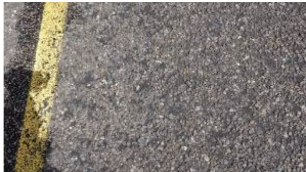
Figure A-341. SH0070-2, Inside WP.
