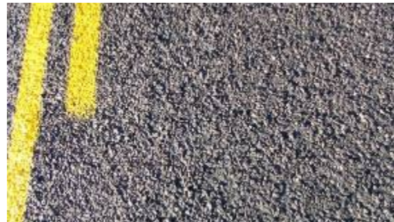
Figure A-896. SH0289-4, Inside WP.
