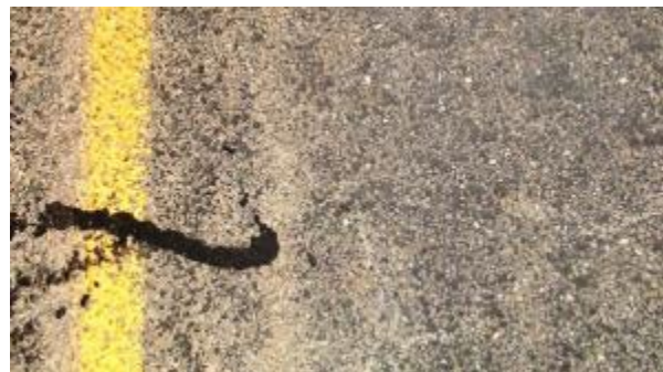
Figure A-36. SH0092-1, Inside WP.
