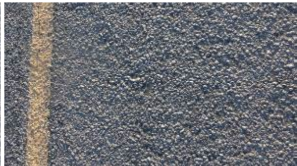
Figure A-92. SH0092-3, Inside WP.
