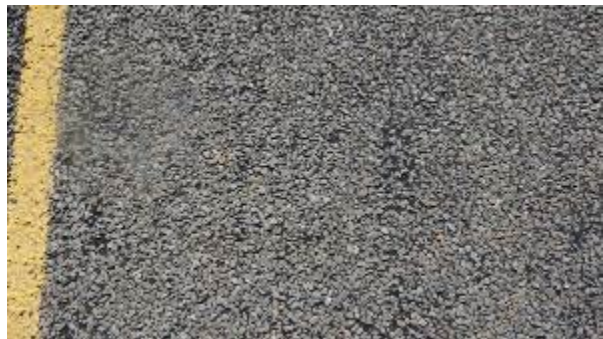
Figure A-513. SH0029-3, Inside WP.
