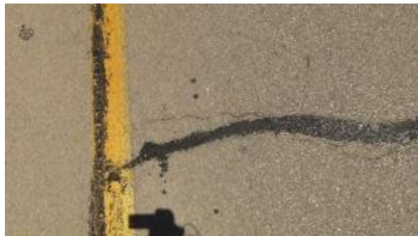
Figure A-44. SH0092-3, Inside WP.
