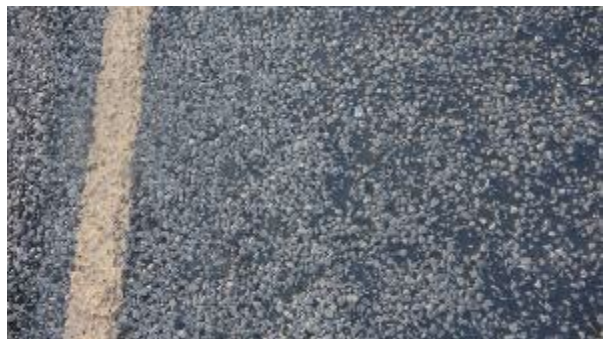
Figure A-84. SH0092-1, Inside WP.
