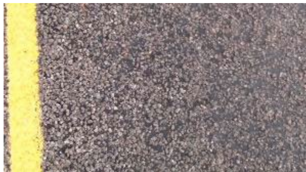
Figure A-52. SH0092-1, Inside WP.
