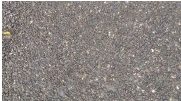
Figure A-357. SH0070-8, Inside WP.
