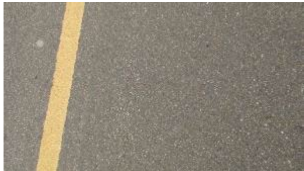
Figure A-333. SH0070-2, Inside WP.
