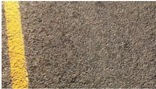
Figure A-72. SH0092-2, Inside WP.
