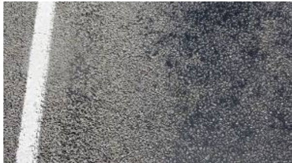
Figure A-549. SH0029-6, Inside WP.
