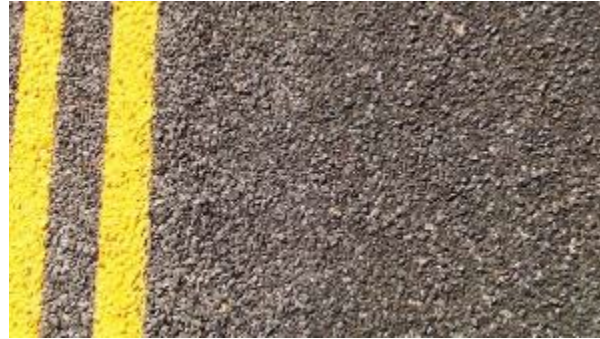
Figure A-64. SH0092-4, Inside WP.
