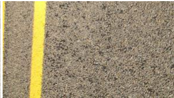
Figure A-489. SH0029-1, Inside WP.
