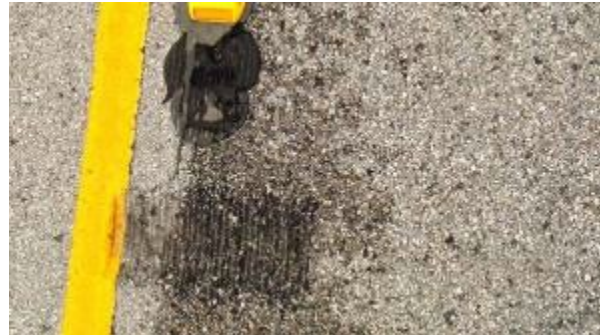
Figure A-868. SH0289-1, Inside WP.
