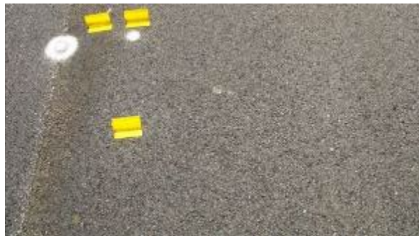
Figure A-465. SH0029-3, Inside WP.
