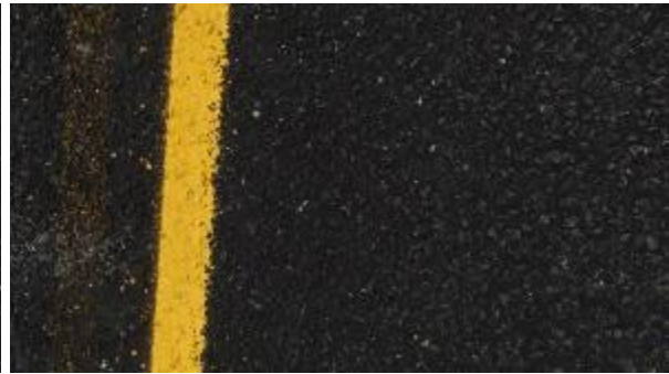
Figure A-906. SH0289-3, Inside WP.
