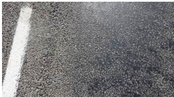
Figure A-545. SH0029-5, Inside WP.
