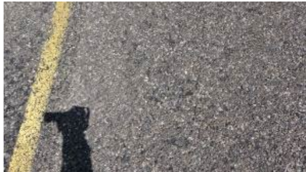
Figure A-373. SH0070-8, Inside WP.
