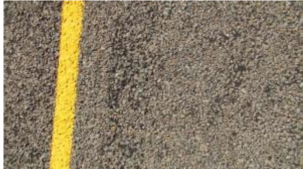
Figure A-501. SH0029-4, Inside WP.
