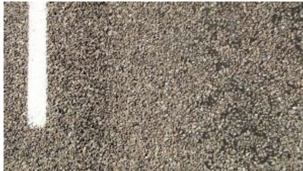
Figure A-533. SH0029-6, Inside WP.
