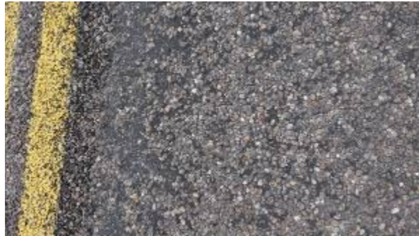
Figure A-337. SH0070-1, Inside WP.
