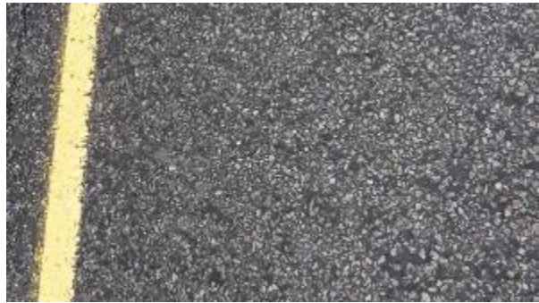
Figure A-922. SH0289-3, Inside WP.
