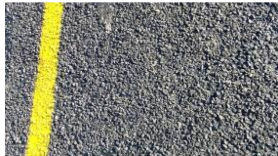
Figure A-892. SH0289-3, Inside WP.
