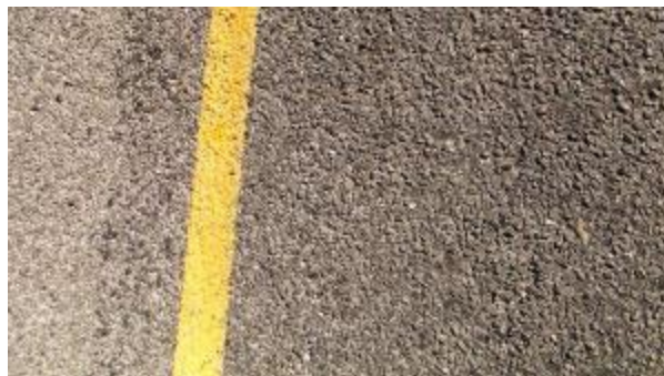
Figure A-76. SH0092-3, Inside WP.
