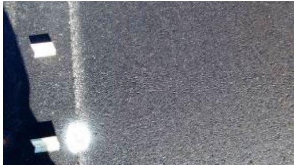
Figure A-525. SH0029-6, Inside WP.
