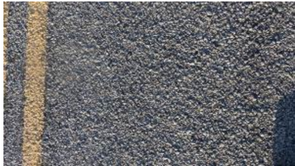
Figure A-96. SH0092-4, Inside WP.
