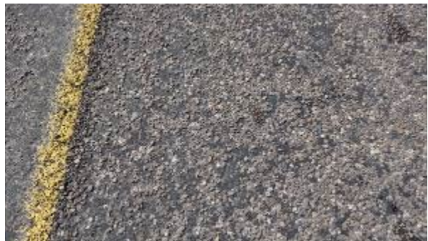
Figure A-361. SH0070-5, Inside WP.
