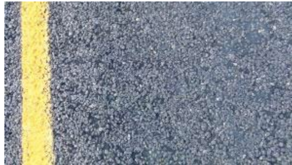
Figure A-56. SH0092-2, Inside WP.
