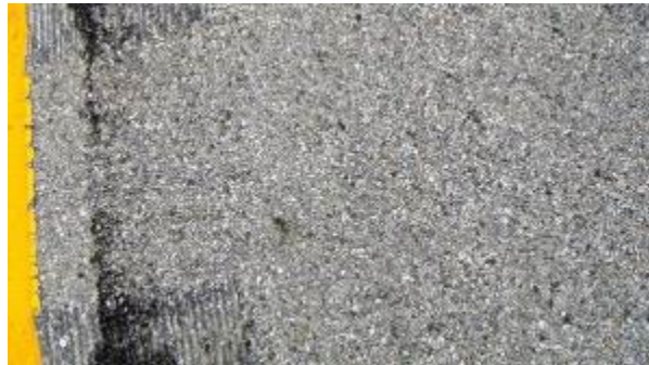
Figure A-880. SH0289-4, Inside WP.
