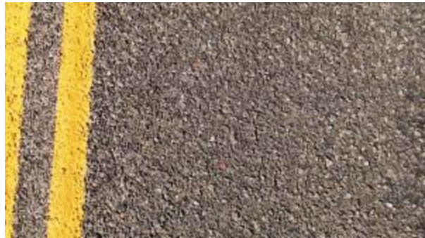
Figure A-80. SH0092-4, Inside WP.
