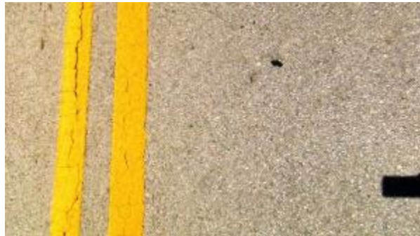
Figure A-48. SH0092-4, Inside WP
