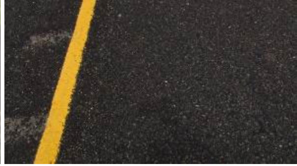
Figure A-902. SH0289-2, Inside WP.
