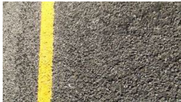
Figure A-60. SH0092-3, Inside WP.
