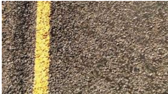
Figure A-68. SH0092-1, Inside WP.
