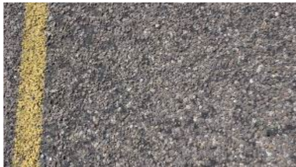
Figure A-369. SH0070-7, Inside WP.
