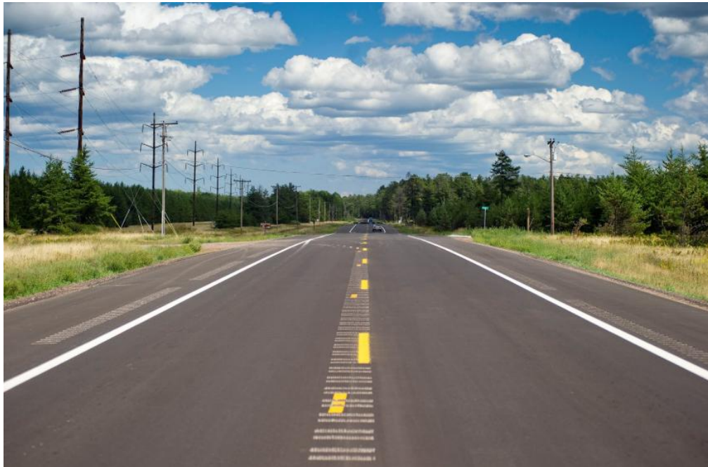
Figure 15. Typical Super 2 Segment with Centerline and Shoulder Rumble Strips.
