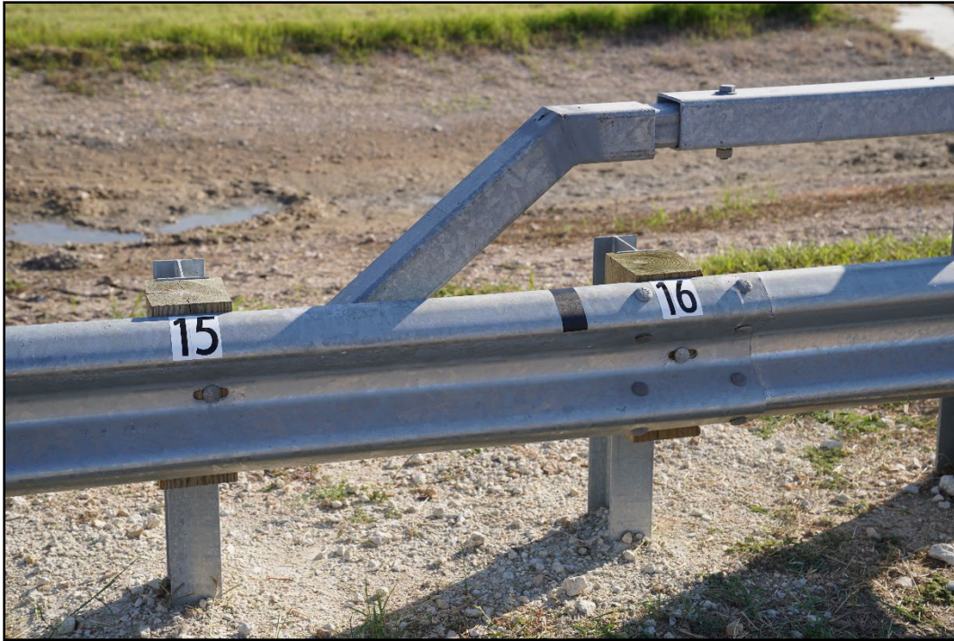
Figure 3.4. TL-4 Test Installation at the Transition Box Beam Rail prior to Testing.
