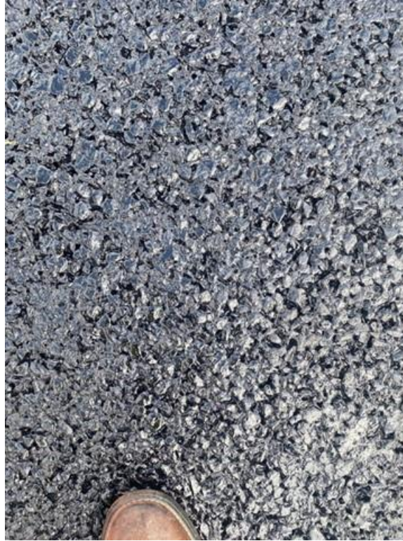
Figure 125. Close-up of fog seal application on PFC.
