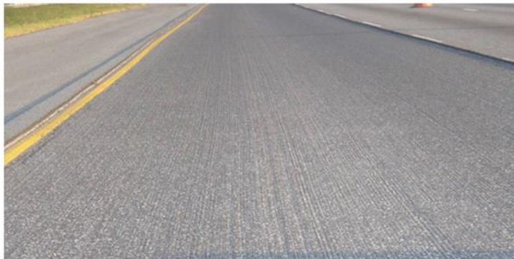
Figure 19. Variable-depth micromilled surface in Georgia (Jared and Hines 2014).
