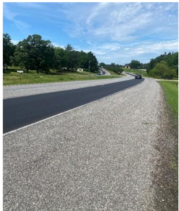
Figure 9. PFC repaired with inlaid, dense-graded hot-mix asphalt since PFC on shoulder was clogged.
