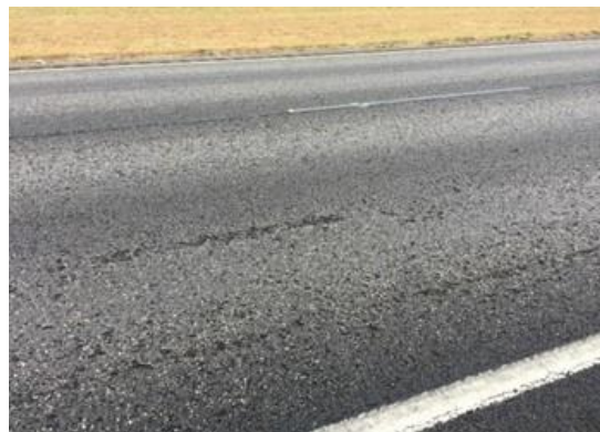
Figure 1. Raveling distress in aged PFC.
