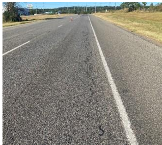
Figure 2. Cracking distress in aged PFC.
