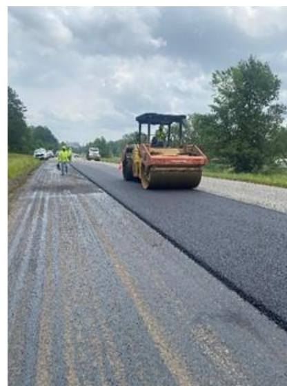
Figure 7. Hot-mix application on PFC.
