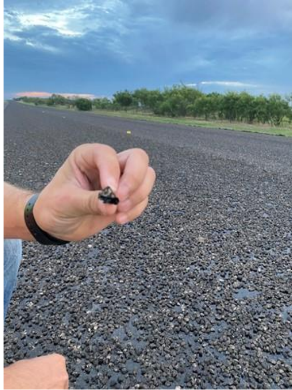
Figure 115. Initial embedment after rolling.
