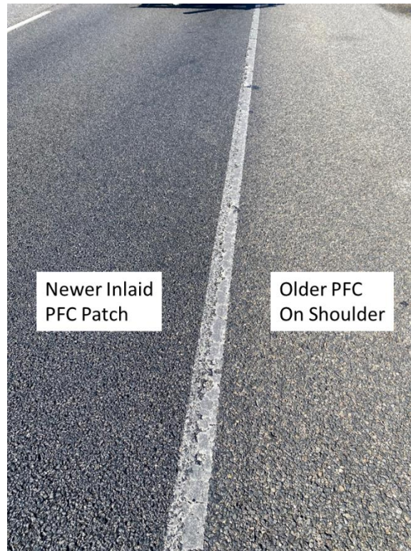
Figure 98. Close-up of newer PFC patch next to older PFC in shoulder.
