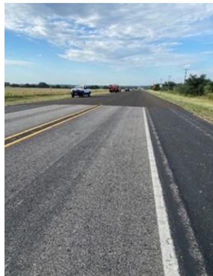
Figure 6. Seal coat application on PFC.
