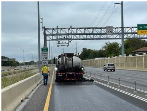
Figure 5. Rejuvenating fog seal application on PFC.
