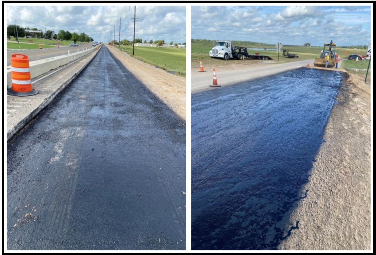
Figure 42. Base Course with Fresh Applied Prime.
