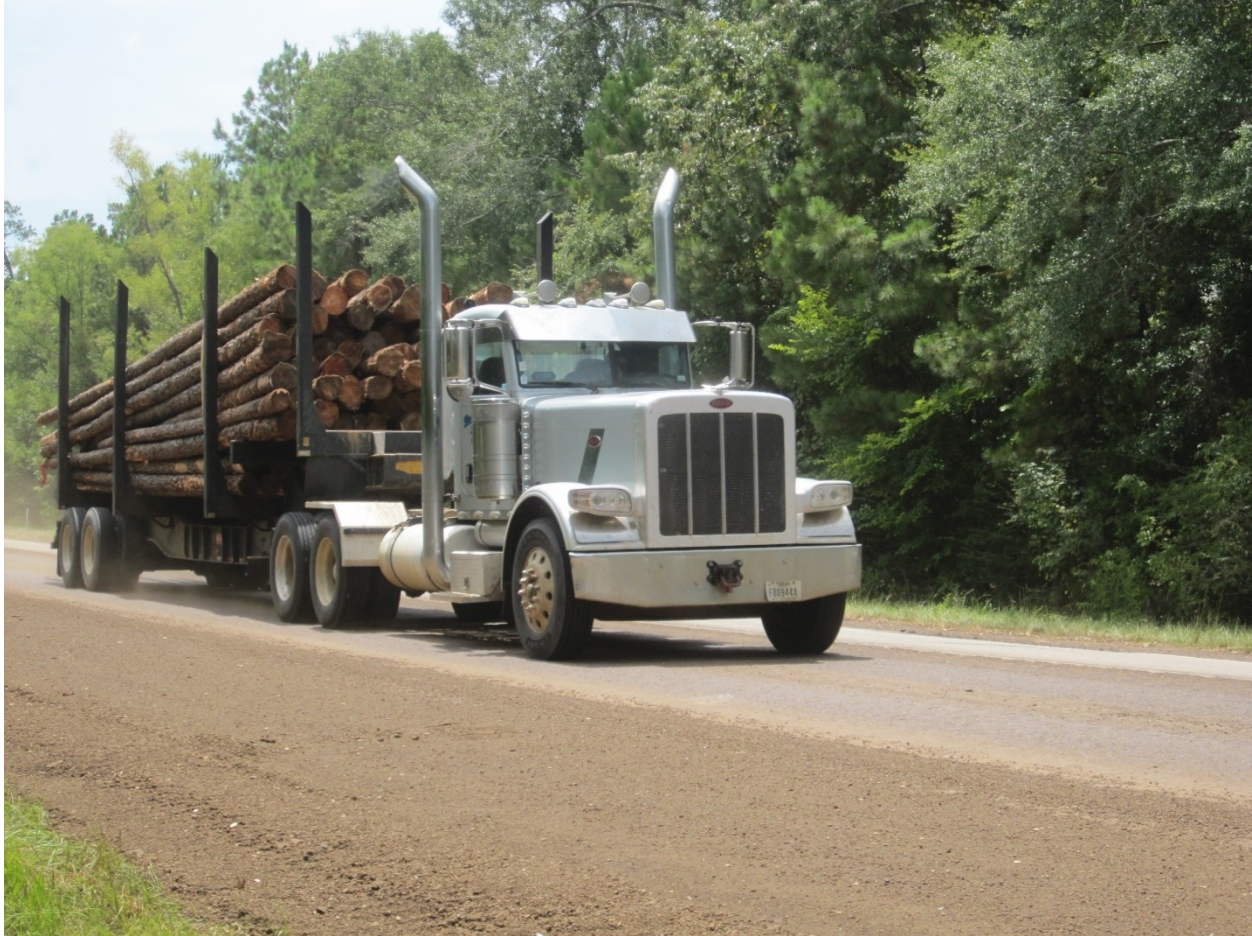
Figure 47. FDR Base Course on US 287 under Traffic prior to Prime.
