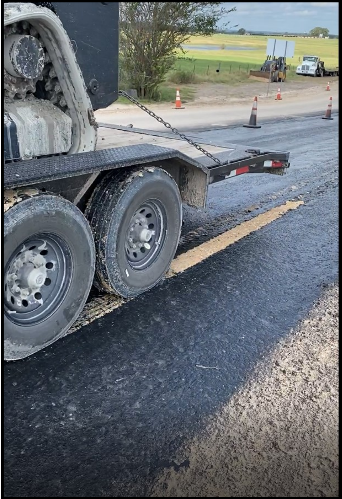
Figure 43. Prime Picking Up on Vehicle Tires.
