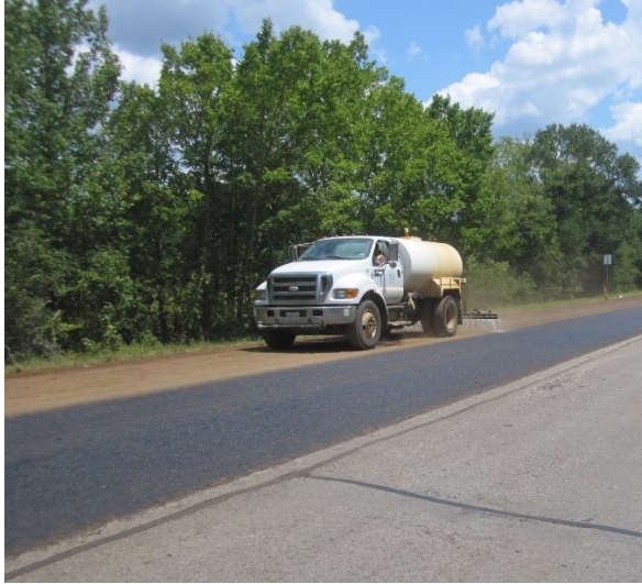
Figure 48. Applying CSS-1H on US 287 FDR Layer.
