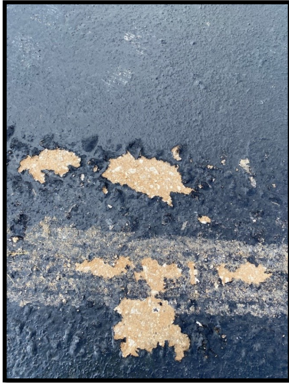
Figure 44. No Penetration of the Prime into the Base.
