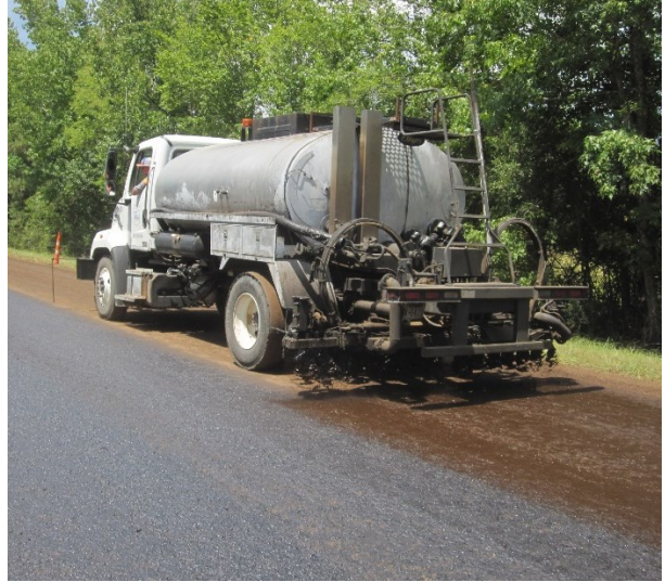
Figure 48. Applying CSS-1H on US 287 FDR Layer.
