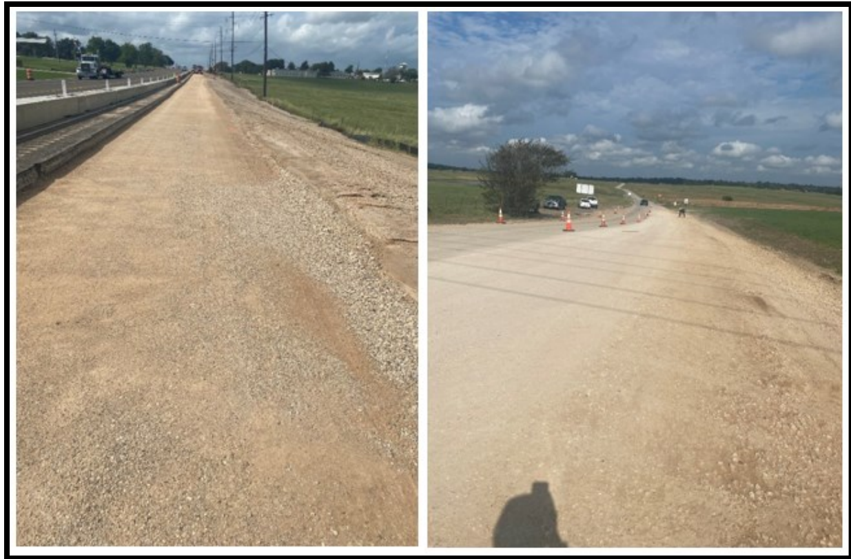
Figure 41. Base Course prior to Priming.
