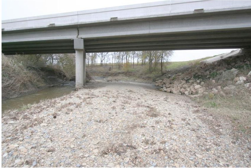
Figure 104. IH 35 NBFR over Cobb Creek Riprap Slope Failure (Courtesy of TxDOT).
