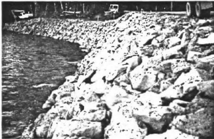
Figure 91. Hoh River at Site 1 Forks Riprap Failure (Blodget & McConaughy, 1986).
