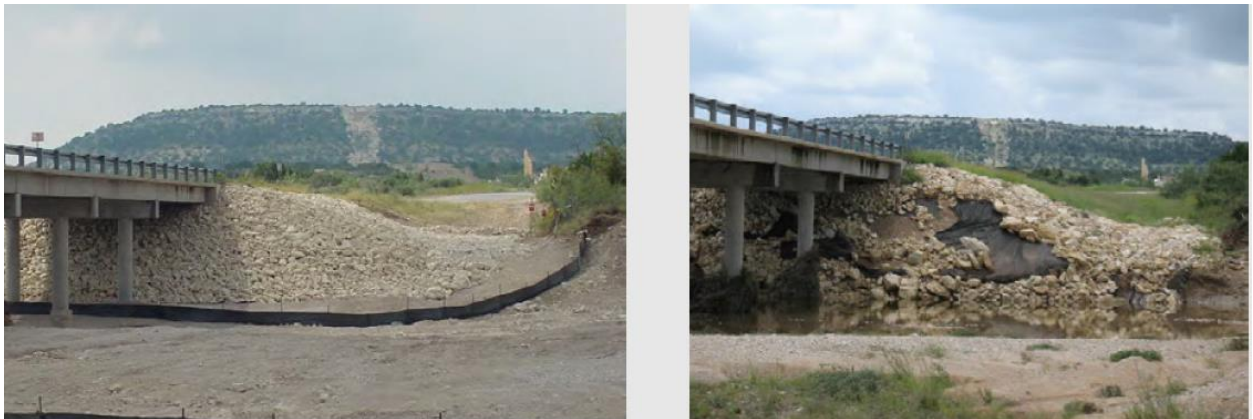
Figure 11. Toe Erosion Slope Failure (Delphia, 2018).
