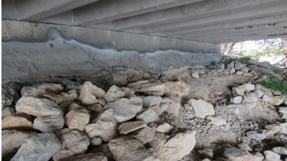
Figure 100. SH 78 over Price Creek Riprap Slope Failure (Courtesy of TxDOT).
