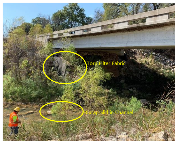
Figure 106. FM 667 Cobb Hollow Riprap Slope Failure (Courtesy of TxDOT).
