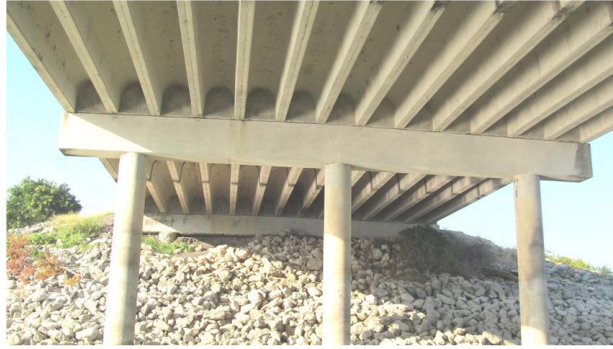
Figure 102. FM 982 over Tickey Creek Riprap Slope Failure (Courtesy of TxDOT).
