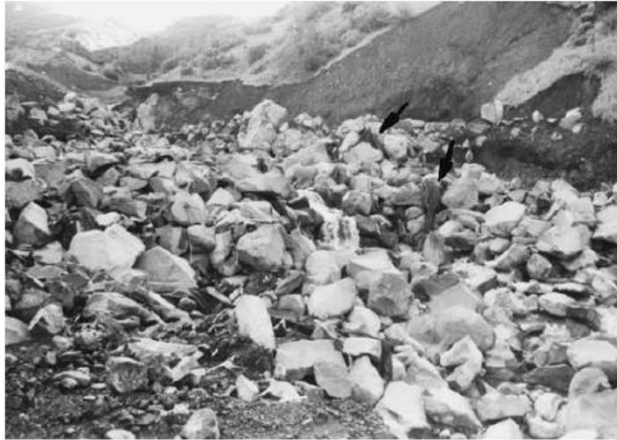
View is looking upstream. Woven-tape geotextile (slit-film) marked with arrows is inappropriate as RSP-fabric on banks (photographed May 1995)
