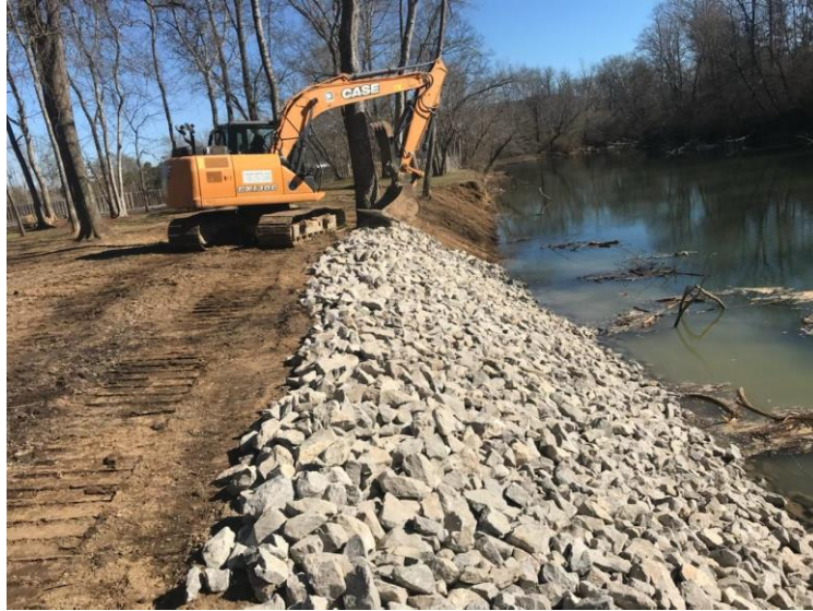
Figure 29. Riprap Installation in Water (Dodd Construction, n.d.).
