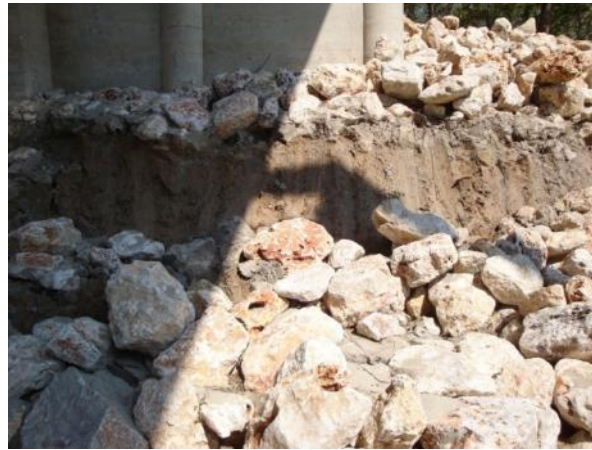
Figure 67. Riprap-Covered Slope Failure (Briaud et al., 2010).
