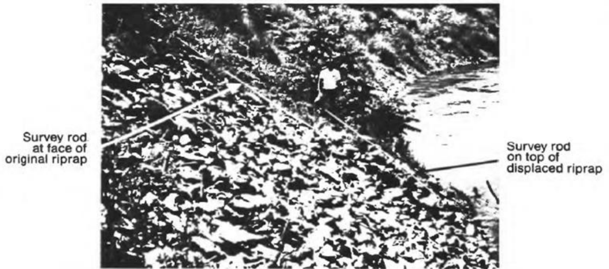
Figure 92. Cosumnes River at Site 3 Riprap Failure (Blodget & McConaughy, 1986).
