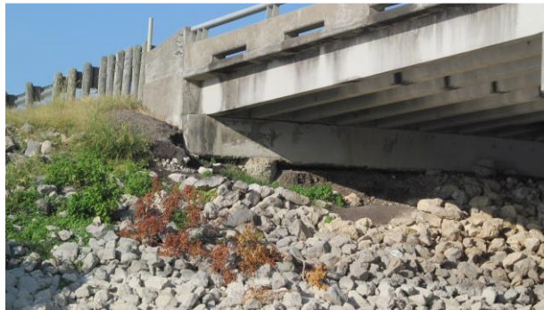
Figure 101. FM 982 over Tickey Creek Riprap Slope Failure (Courtesy of TxDOT).
