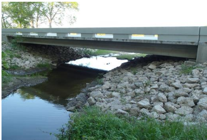
Figure 97. FM 1155 Little Sandy Creek Riprap Failure (Courtesy of TxDOT).
