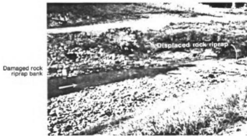
Figure 89. Pinole Creek Riprap Failure (Blodget & McConaughy, 1986).
