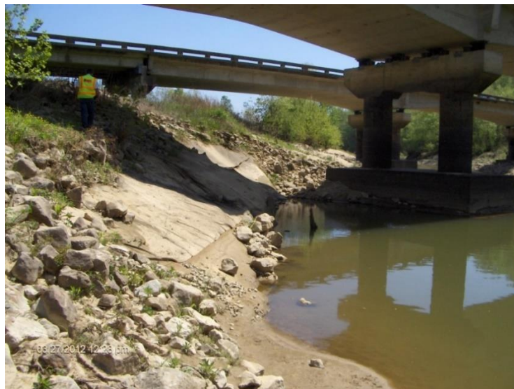
Figure 87. Riprap Slope Failure (Courtesy of Mississippi DOT).
