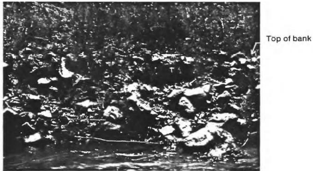
Figure 93. Truckee River at Sparks Riprap Failure (Blodget & McConaughy, 1986).
