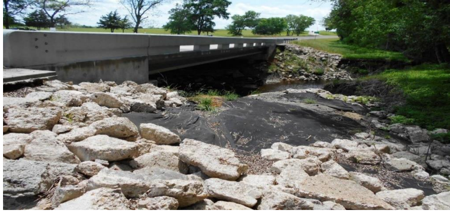
Figure 98. Geotextile underneath the Riprap (Courtesy of TxDOT).
