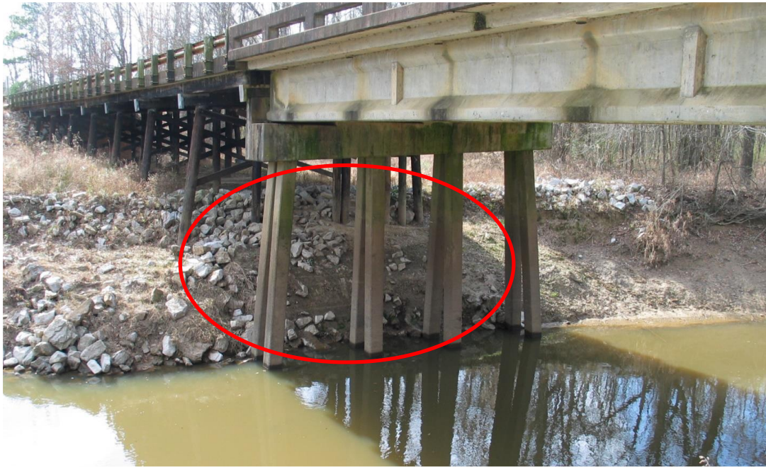
Figure 88. Riprap Slope Failure (Courtesy of Mississippi DOT).
