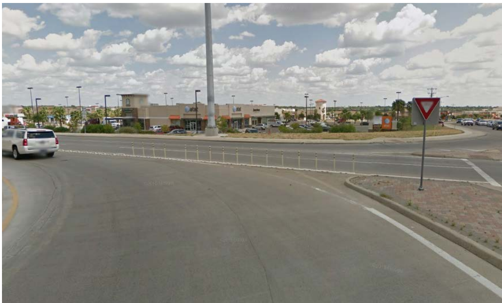
Figure 25. U-Turn Departure Installation of Pylons.
