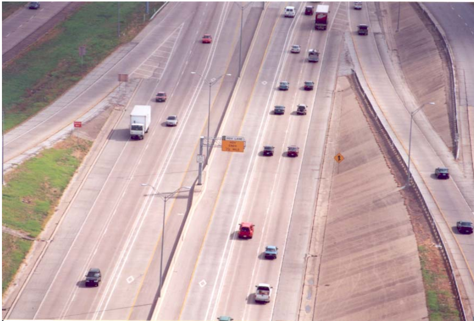
Figure 9-16. HOV Lane Pavement Marking Symbols in Houston.
