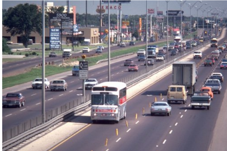
Figure 2-4. IH-45 (North) Contraflow HOV Lane, Houston, Texas (5).
