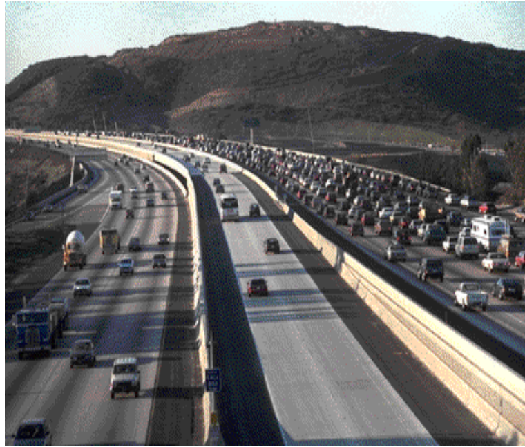
Figure B-1. IH-15 in San Diego, California.
