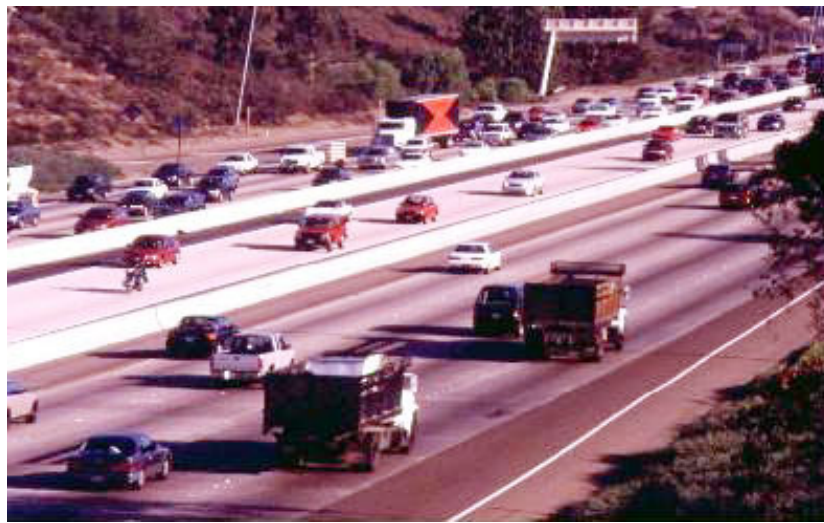
Figure 2-6. IH-15 HOV/HOT Lanes, San Diego, California (5).
