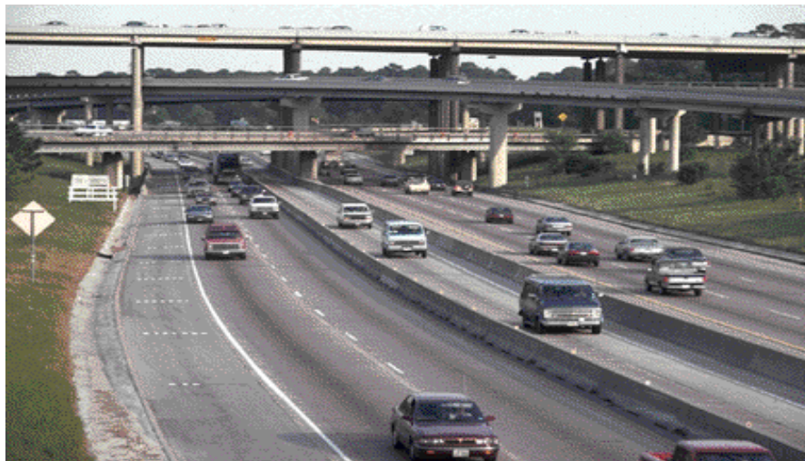
Figure B-2. IH-10 Katy Freeway in Houston, Texas.
