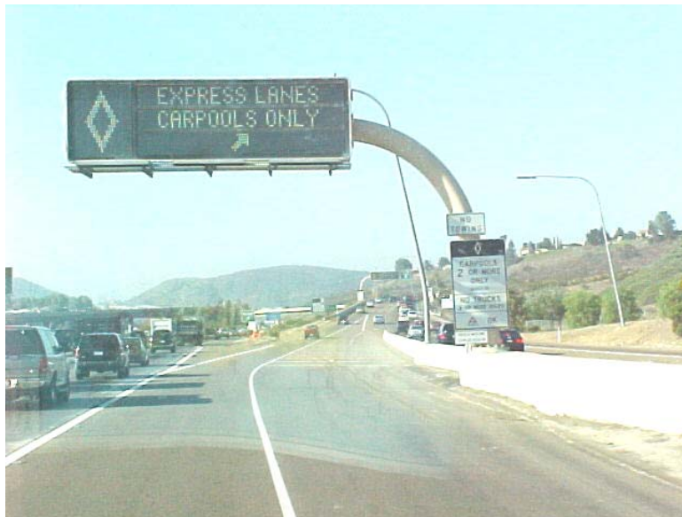
Figure 9-15. Overhead Dynamic Message Sign.
