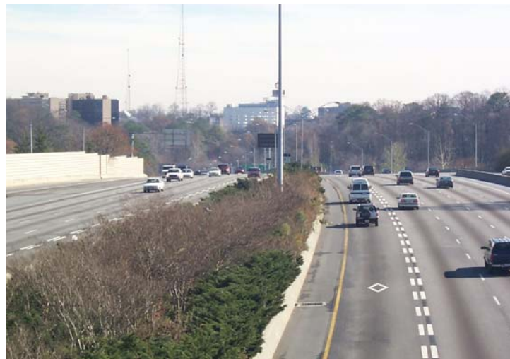
Figure 2-5. IH-75 Contraflow HOV Lane, Atlanta, Georgia (5).
