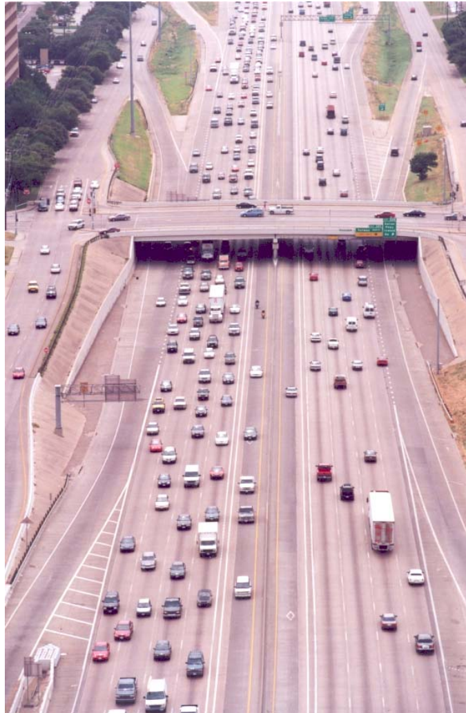
Figure 2-3. IH-635 (LBJ) Concurrent-Flow, Buffer-Separated HOV Lane, Dallas, Texas.
