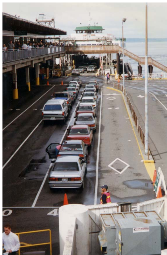
Figure 2-11. HOV Queue Bypass, Coleman Dock Ferry, Seattle, Washington (5).
