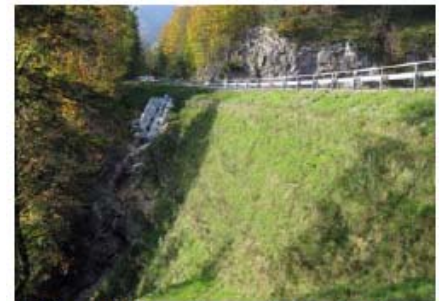
Reinforced fill slope 2 years after construction
