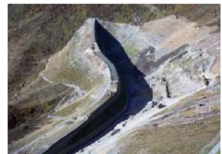
Avalanche protection barrier almost completed
