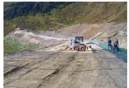
Miragrid® GX geogrid reinforcement being placed in the reinforced slope
