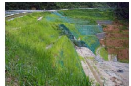
Completed reinforced slope with vegetation being established
