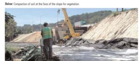
Below: Compaction of soil at the face of the slope for vegetation.
