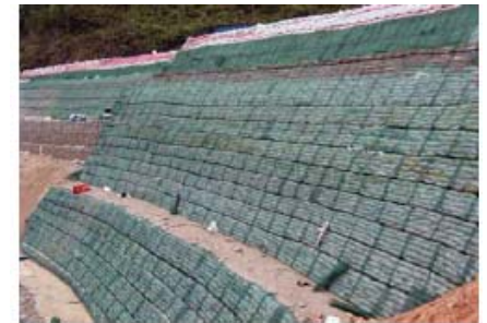
Reinforced slope partially completed
