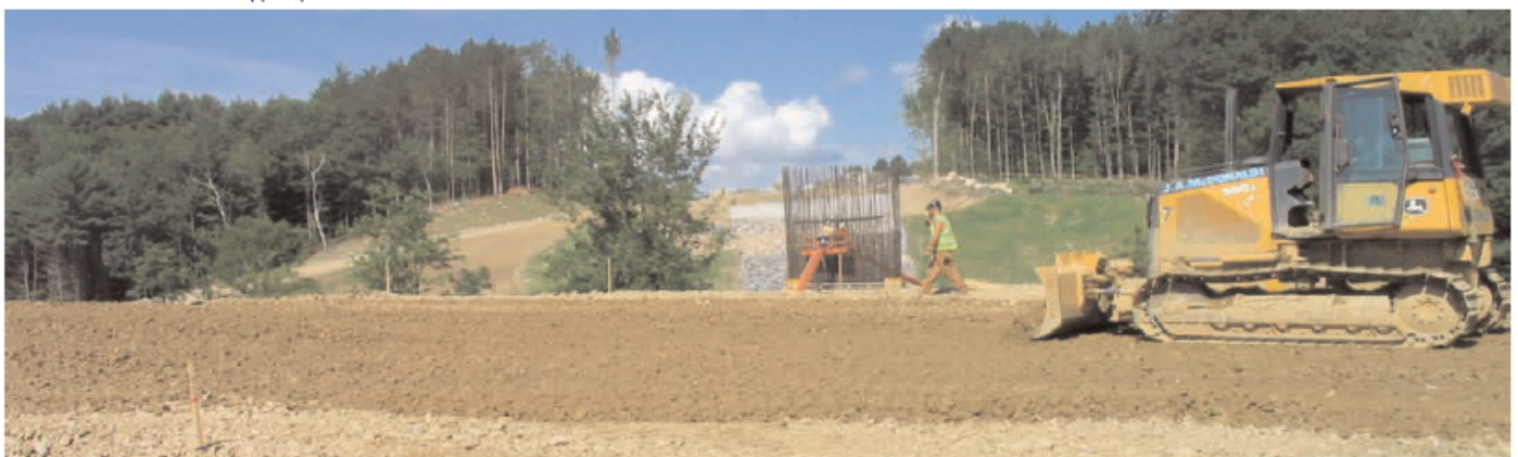
BELOW: Final elevation of support pad for west abutment.
