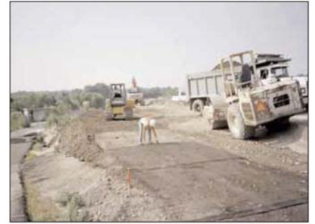
Miragrid* BXT, used as the primary reinforcement, is installed in 0.9 m (3.0 ft) embedment lengths.
