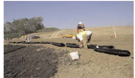
Pre-cut lengths of 21m (69ft) Miragrid® 10XT geogrid ready to be rolled out.
