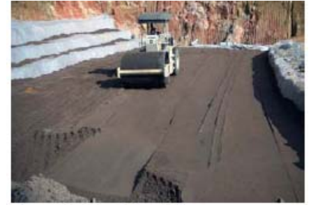
Compacting the reinforced fill
