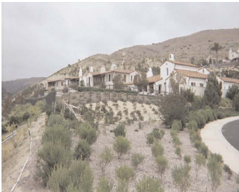
These premium lots were considered unbuildable. Miragrid® geogrids made it possible to develop this valuable property.
