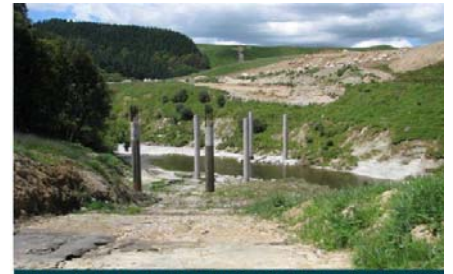
Bridge prior to construction with piers installed Date: Feb 2009
