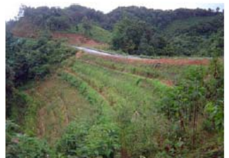
Completed reinforced slope with vegetation growth on the face
