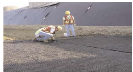
Installing stakes to keep geogrid positioned.
