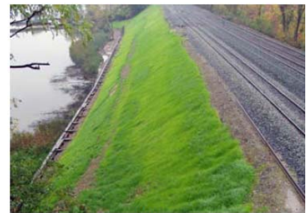
Completed reinforced fill slope with vegetated surface
