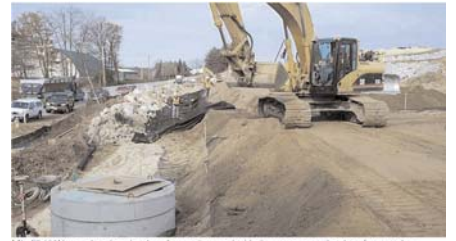
Miragrid® 180N was placed on the slope face and covered with riprap to protect the slope from erosion.
