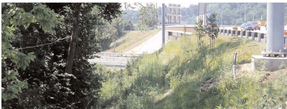
Completed slope with vegetation.
