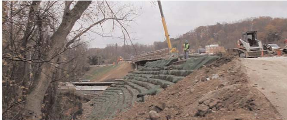
Slope nearing the finished grade.
