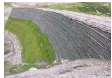
Wire mesh facing on the reinforced slope face with vegetation applied to the lower part of the slope
