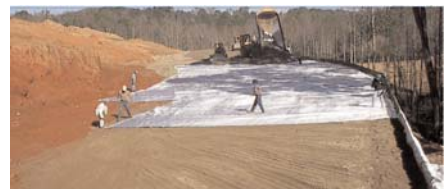
To complete this reinforced slope, 44,723m 2 (53,500yd 2 ) of the HS400PP and 43,495m 2 (56,000yd 2 ) of the HS800PP were installed as primary reinforcement.
