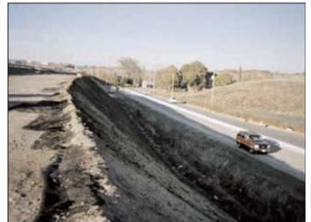
The 2:1 MSE slope at Marston Street was steepened to 1:1.
