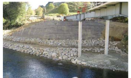
Completed Green Terramesh abutment structure Date: April 2009
