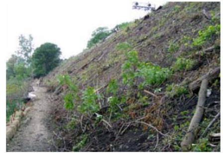
Clearing of vegetation from the existing embankment slope
