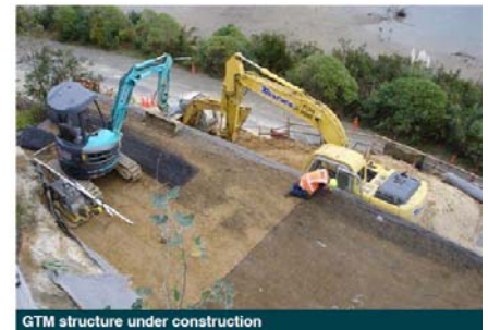
GTM structure under construction
