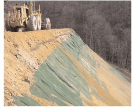
Early construction at the bottom of the slope.
