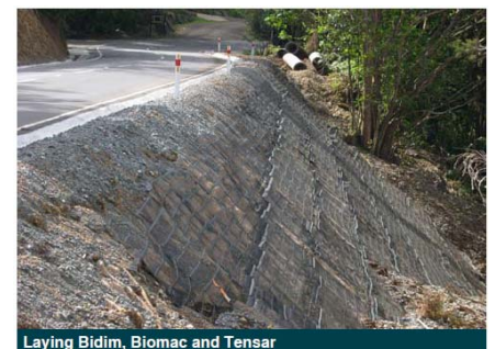
Laying Bidim, Biomac and Tensar
