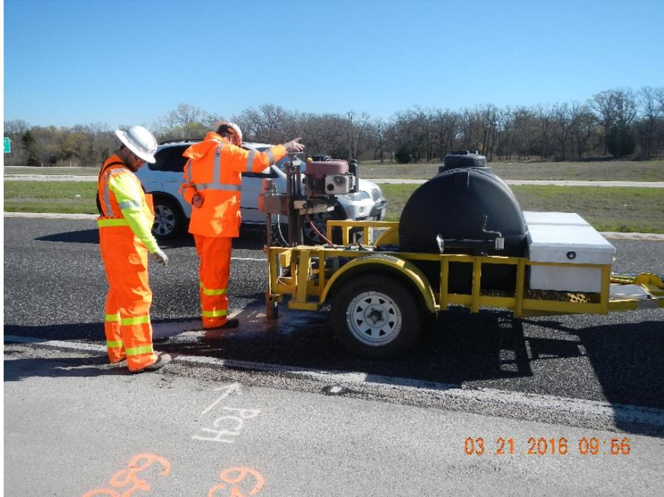
**Figure 3.8 Coring operation**
