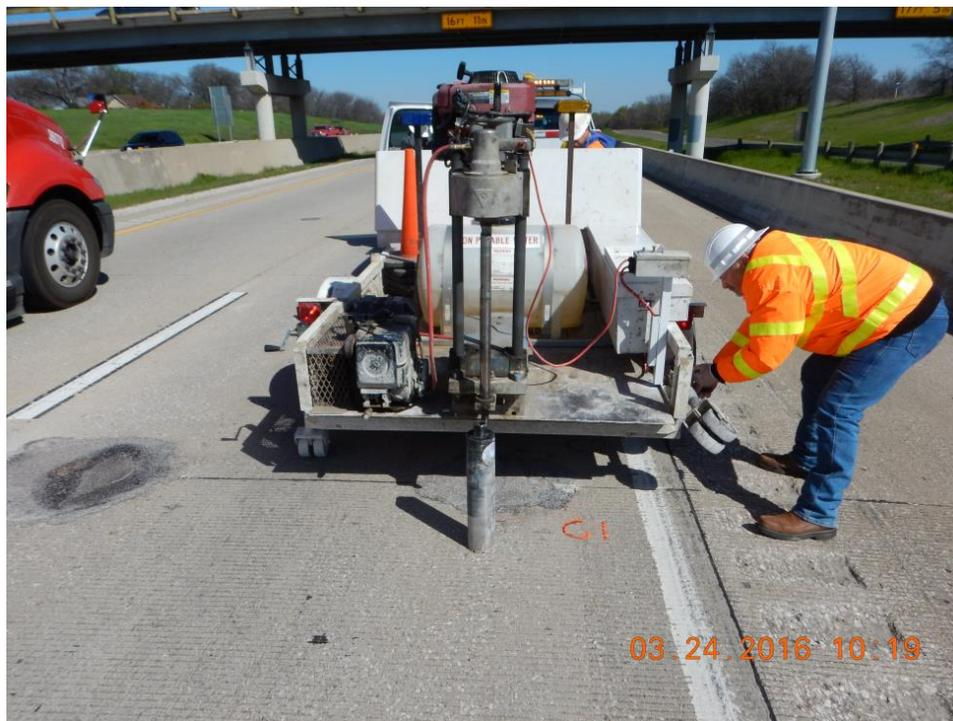
**Figure 3.54** Coring operation on IH 35 in Denton County
