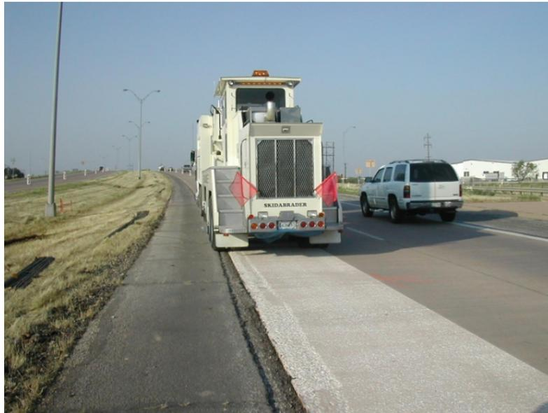
(a) Shot-blasting operation of the concrete surface
