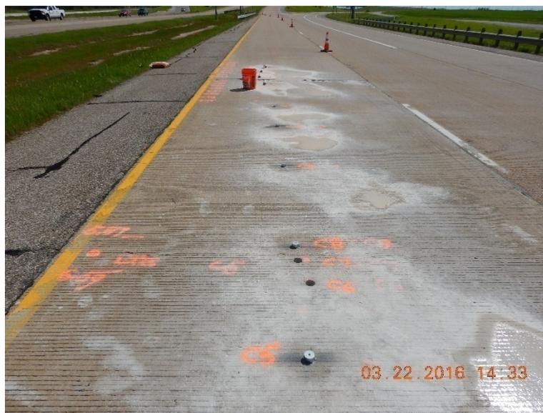
**Figure 4.8 Bond strength testing on US 281 in Wichita Falls**
