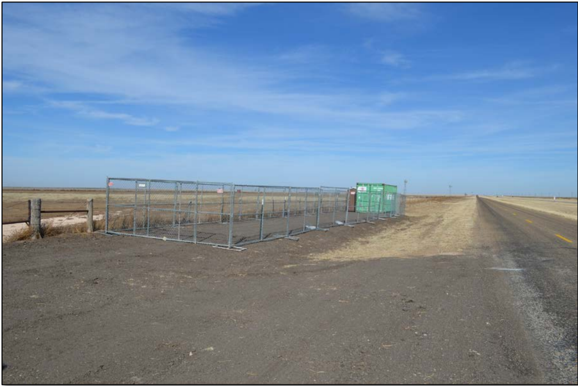
Figure 2.12. Field Site Enclosure, South End, Field Test Site 4a, Randall County, TX
