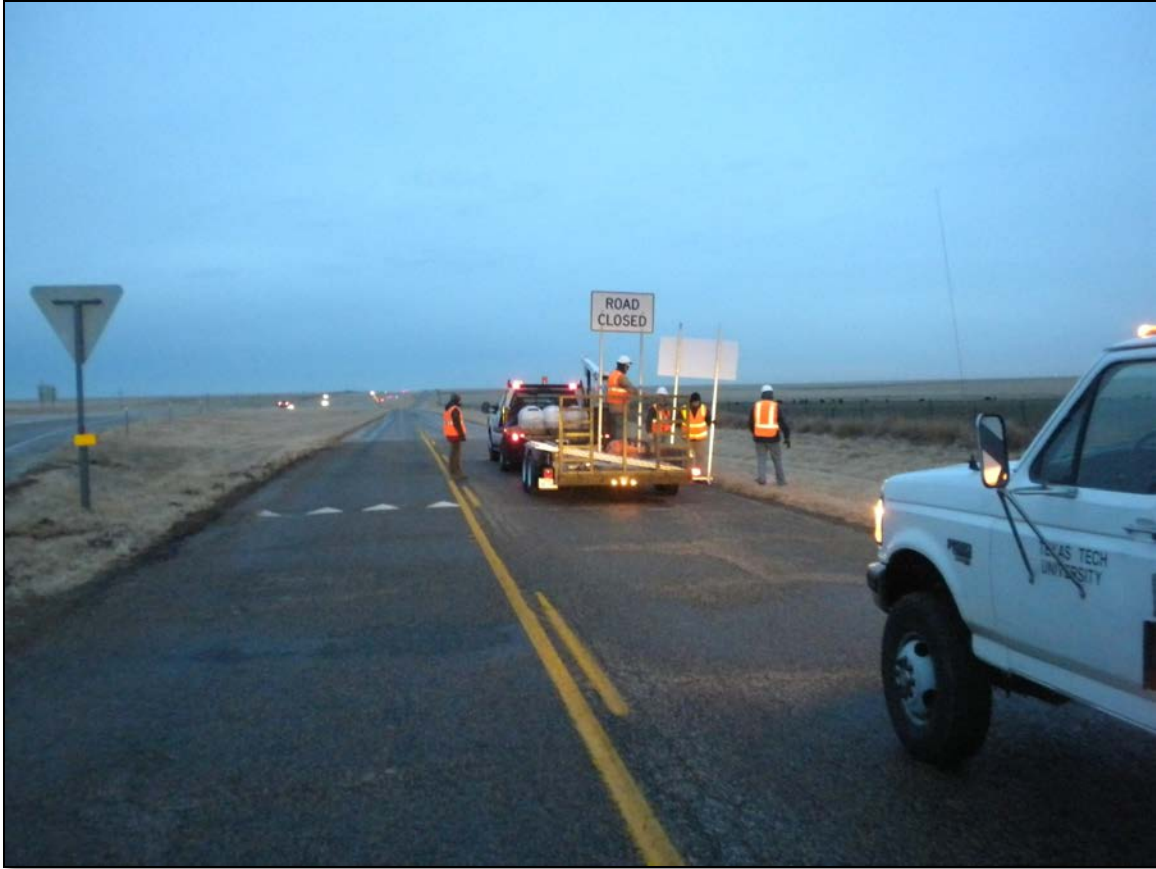
Figure 2.20. Deploying Traffic Control Signage for Road Closure, Storm Event 1, 12/20/2013
