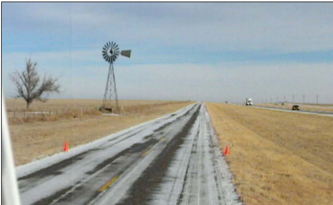
Figure 3.4. Clearing pavement surface condition (still image from video capture)
