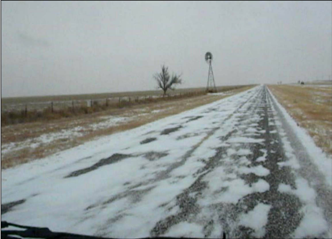
Figure 4.4. Very Cold Temps, Dry Powdery Snow, Variable Snow Accumulation on Road Surface Prior to Storm Event 2-2
