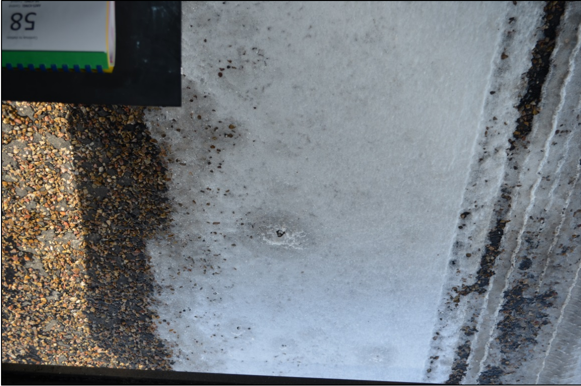
Figure 3.12. Treated Pavement with Melting Snow
