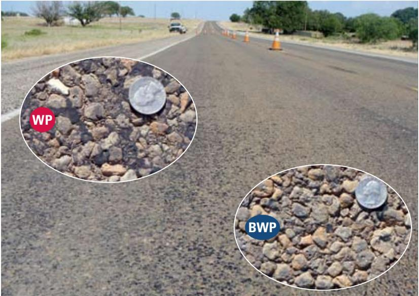
Figure 5. Lane with Mild Flushing.
