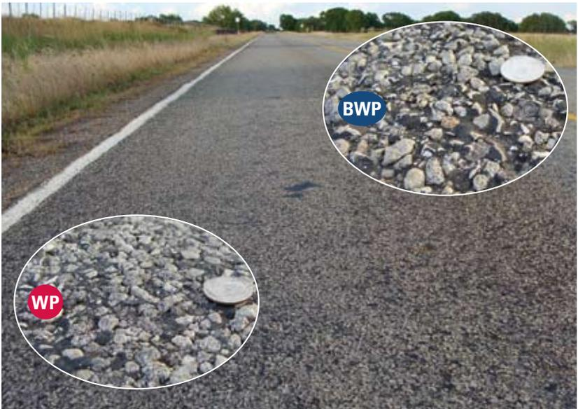
Figure 6. Lane with Slight Wheel Path Color Difference.
