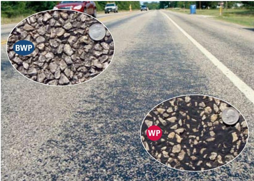
Figure 3. Lane with Moderate Flushing.
