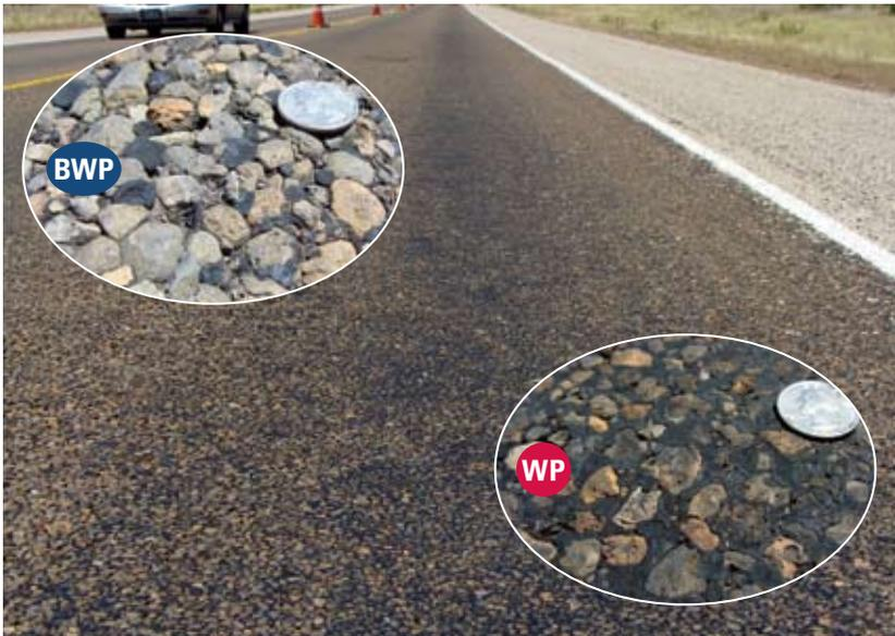
Figure 4. Lane with Mild to Moderate Flushing.
