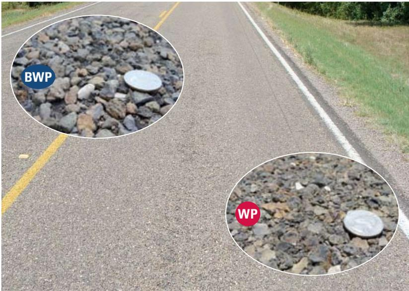
Figure 7. Lane with No Wheel Path Color Difference.
