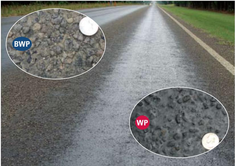
Figure 2. Lane with Moderate to Severe Flushing.
