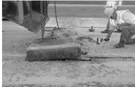
2. Slab removal
