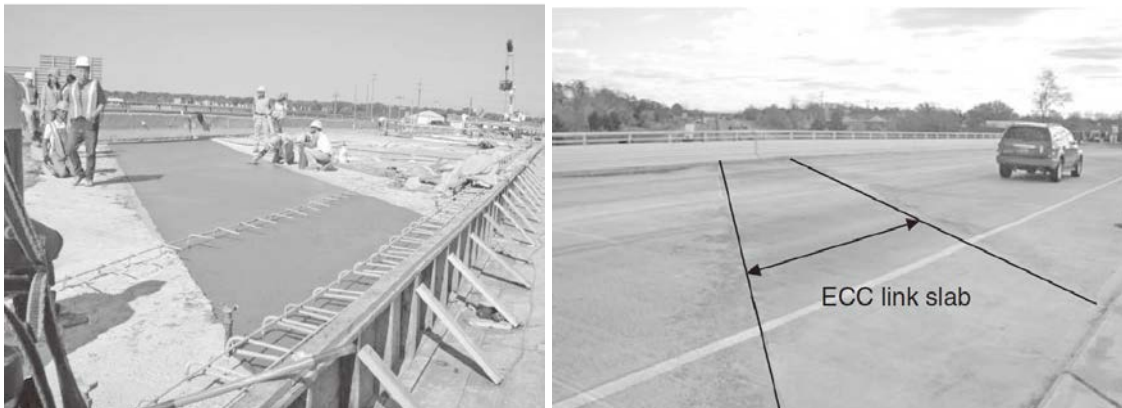
Figure 5-4 ECC Link Slab Constructed in Michigan (Li 2014)
