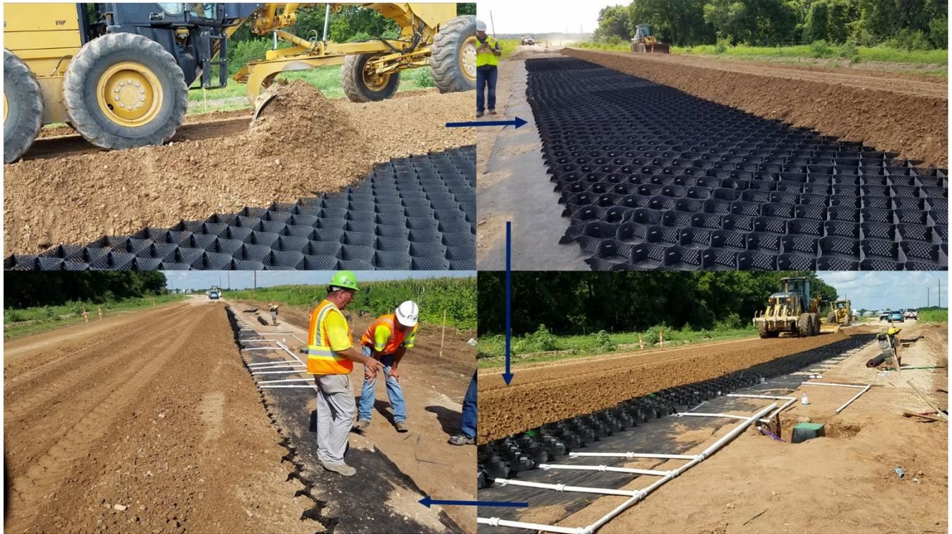
**Figure A-22 Geocell Construction Sequence.**
