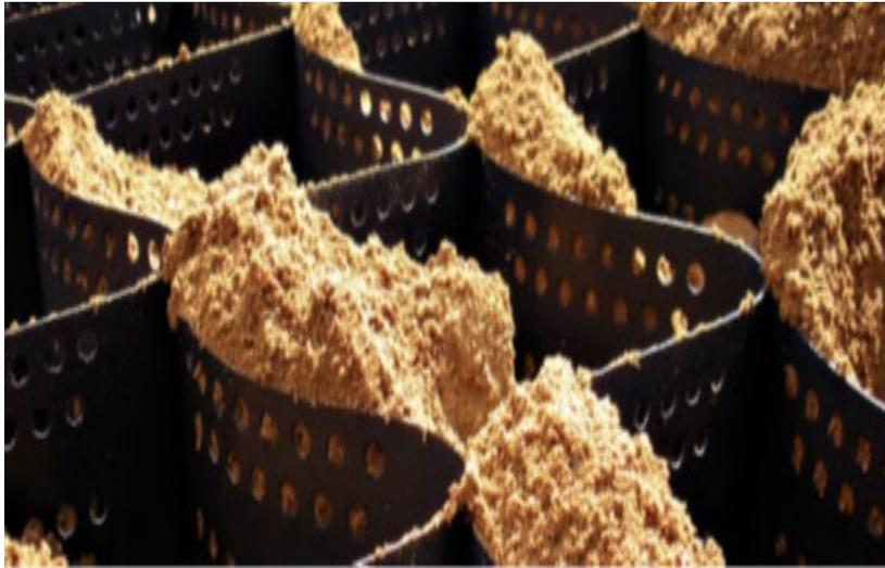
**Figure B-1 Geocell and Infill Material.**
