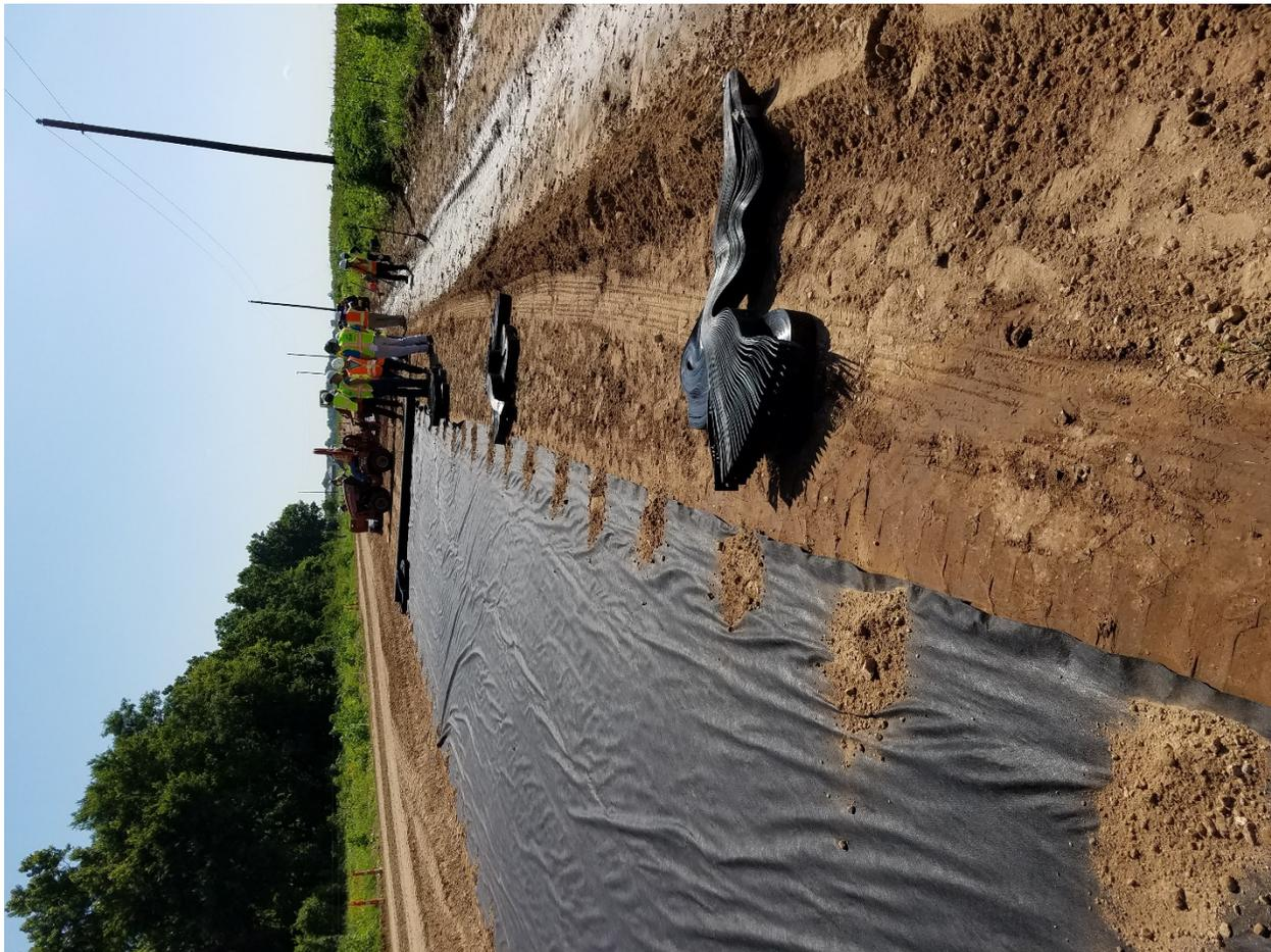
**Figure A-20 Installation of Geosynthetics.**
