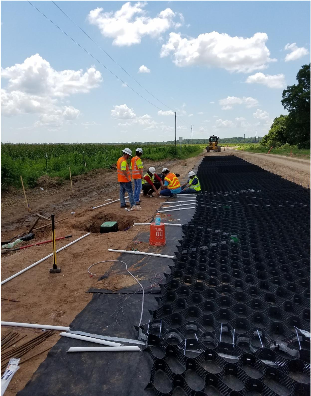
**Figure A-21 Installation of Instrumented Geocells.**
