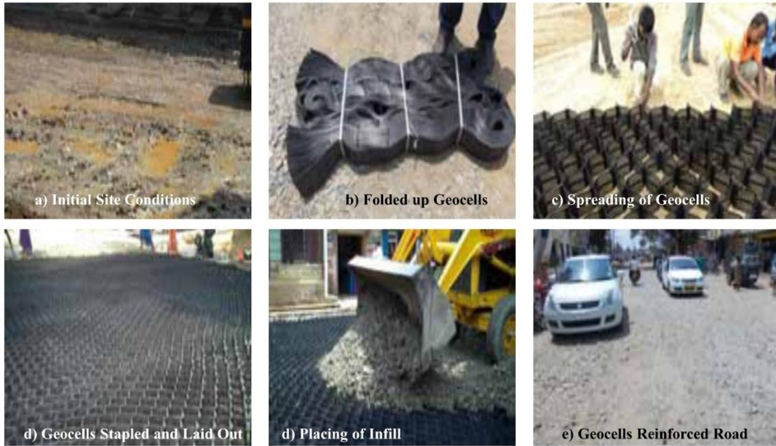
**Figure 2-3 Geocell Construction Sequence.**
