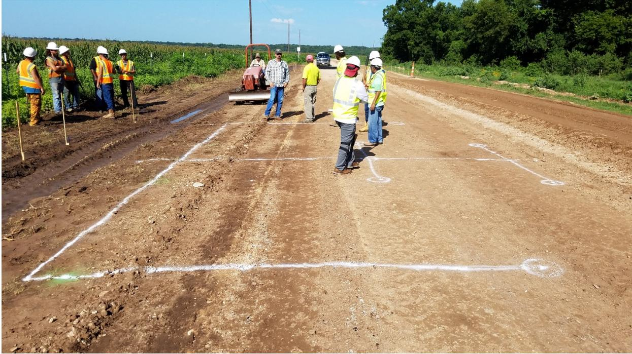
**Figure A-18 Marked Sensor Location for Unreinforced Section.**
