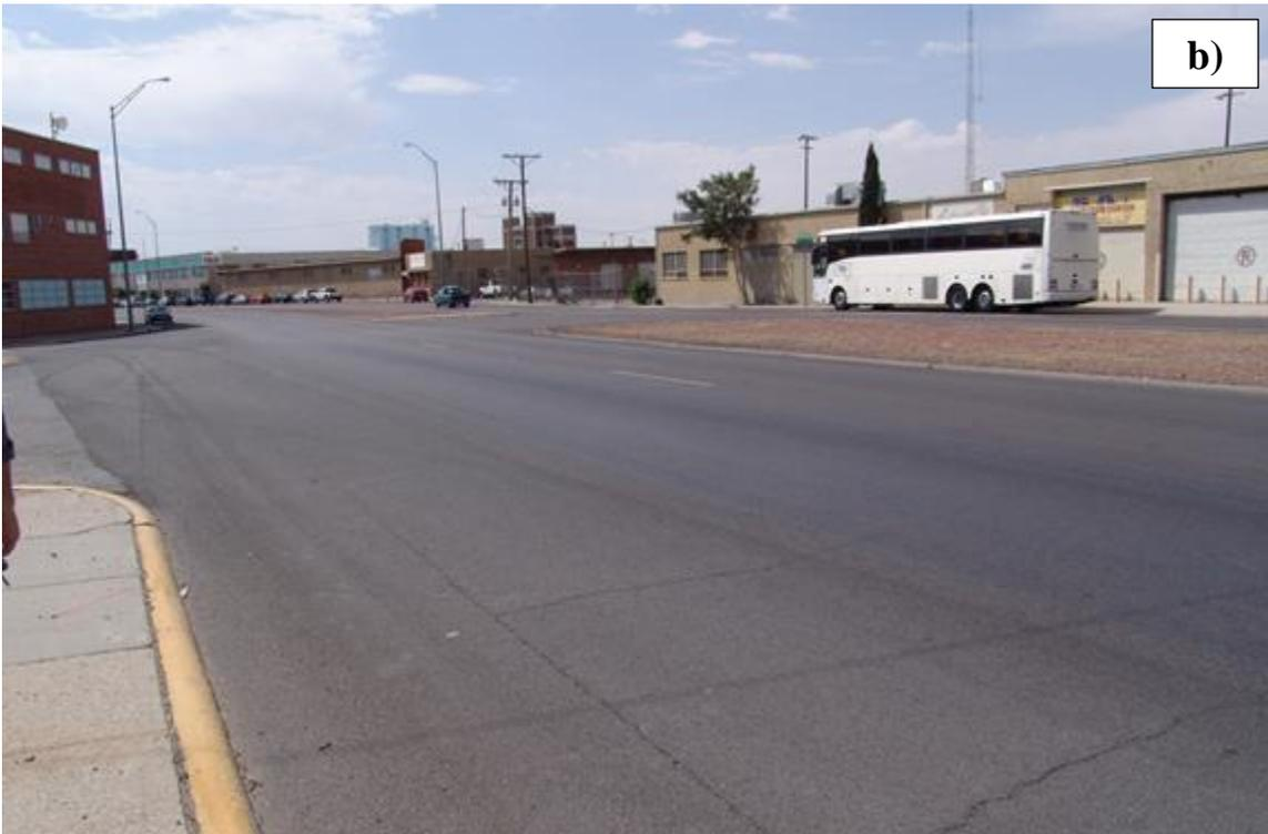
**Figure D27 - Section Condition for Section 16: a) View of Pavement Section and b) Typical Cracking Distress**
