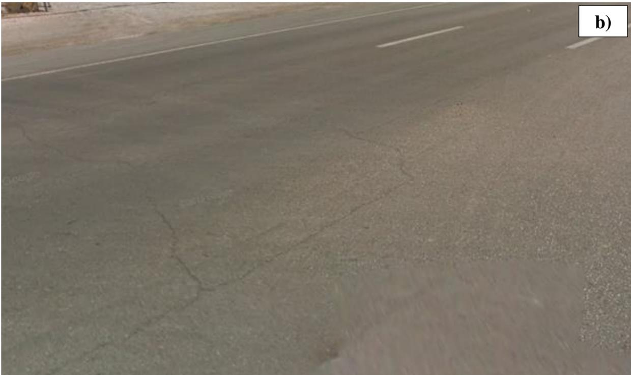
**Figure D25 - Section Condition for Section 14: a) View of Pavement Section and b) Typical Cracking Distress**
