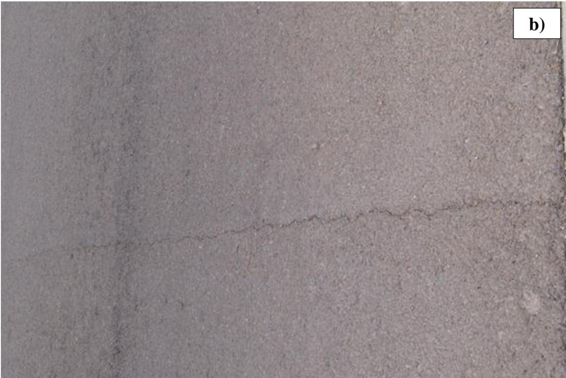
**Figure D21 - Section Condition for Section 10: a) View of Pavement Section and b) Typical Cracking Distress**
