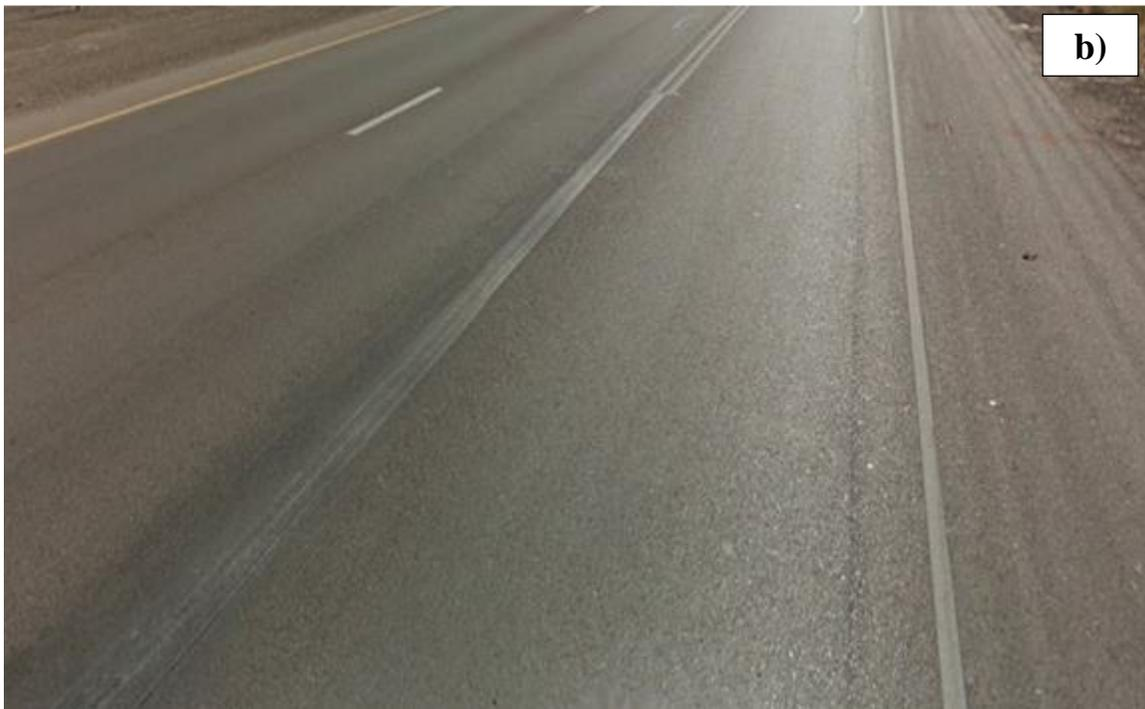
**Figure D24 - Section Condition for Section 13: a) View of Pavement Section and b) Typical Cracking Distress**
