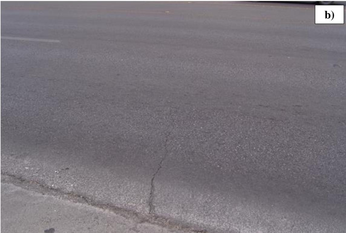
**Figure D22 - Section Condition for Section 11: a) View of Pavement Section and b) Typical Cracking Distress**
