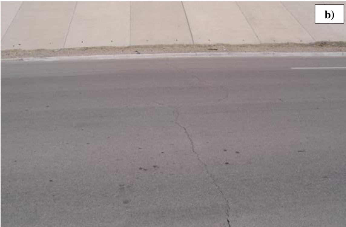
**Figure D20 - Section Condition for Section 9: a) View of Pavement Section and b) Typical Cracking Distress**
