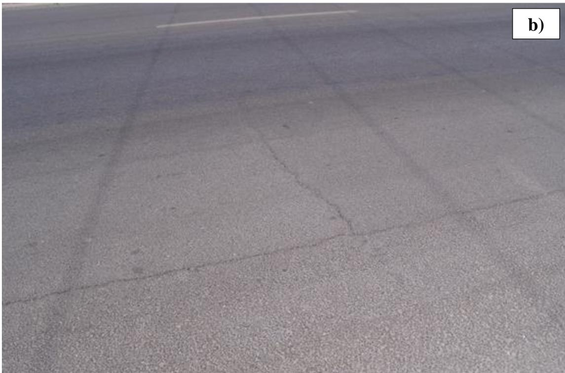
**Figure D28 - Section Condition for Section 17: a) View of Pavement Section and b) Typical Cracking Distress**
