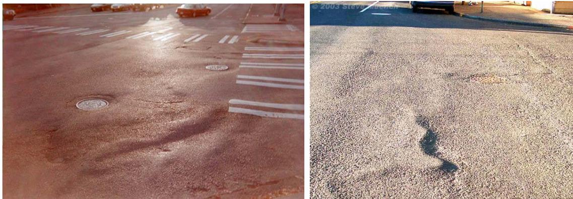
**Figure 2.6 - Shoving on Asphalt Pavements.**
