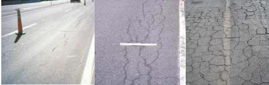
**Low Severity:** Few connecting cracks with no spalling; cracks are not sealed.
