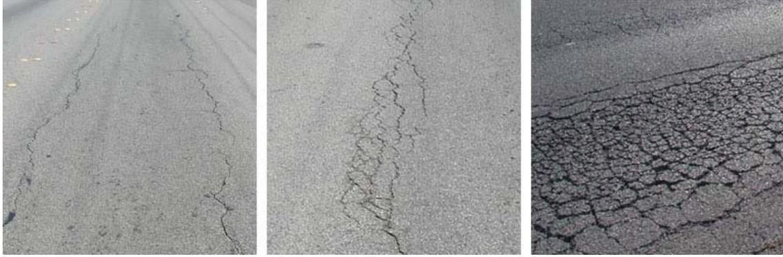
**Figure 2.7 - Fatigue or Alligator Cracking on Asphalt Pavements.**
