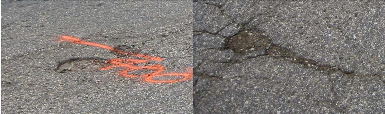
**Figure 5.6 - Cracking Resulting in Potholes on SH 49.**
