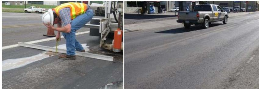
**Mechanism:** Excessive vertical compressive stresses on the HMA surface causing non-recoverable permanent deformation in the asphalt layer of a pavement structure. Surface rutting will be classified to three levels of severity: a) Low severity is measured less than 0.5 in., b) Medium severity is measured greater than or equal to 0.5 in. and less than 1 in. and c) High severity is measured greater than or equal to 1in.
