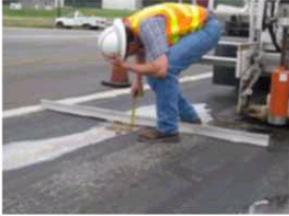
**Mechanism:** Excessive vertical compressive stresses on the HMA surface causing non-recoverable permanent deformation in the asphalt layer of a pavement structure. Surface rutting will be classified to three levels of severity: a) Low severity is measured less than 0.5 in., b) Medium severity is measured greater than or equal to 0.5 in. and less than 1 in. and c) High severity is measured greater than or equal to 1in.
