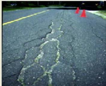
The cracking in the subgrade induced by the shrinkage strain is initiated at a moisture content of 21.60%
