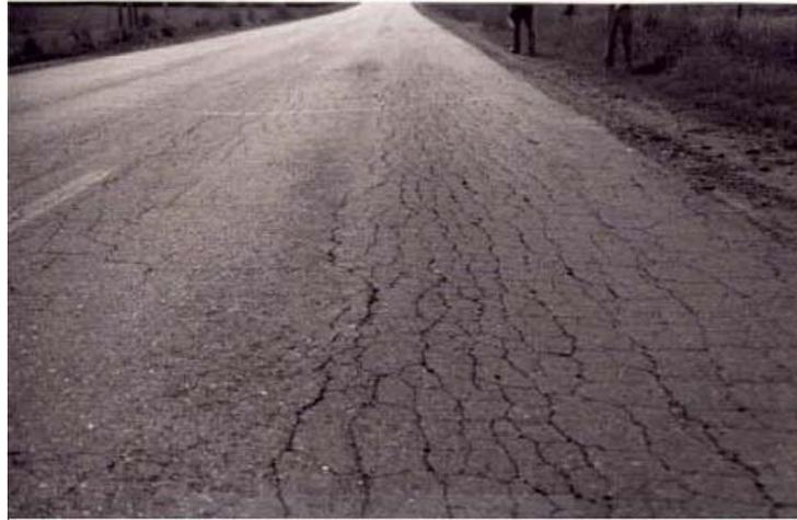
**Figure 2.2 – Distortion and Cracking of Pavements**
