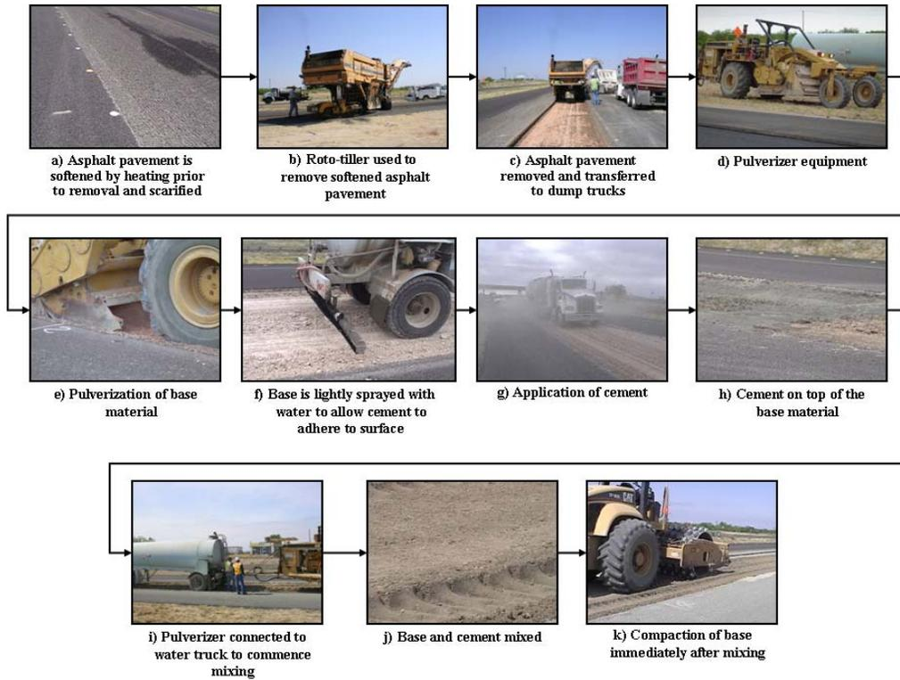
**Figure 4.1 – Construction Procedure used for I-10, and I-20**
