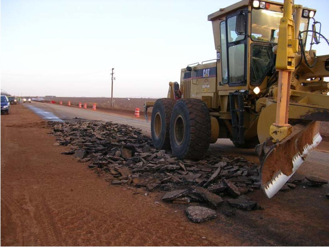
**Figure 5.1 – Hot Mix/Surface-Treatment Layer Retrieved from the Construction Site**
